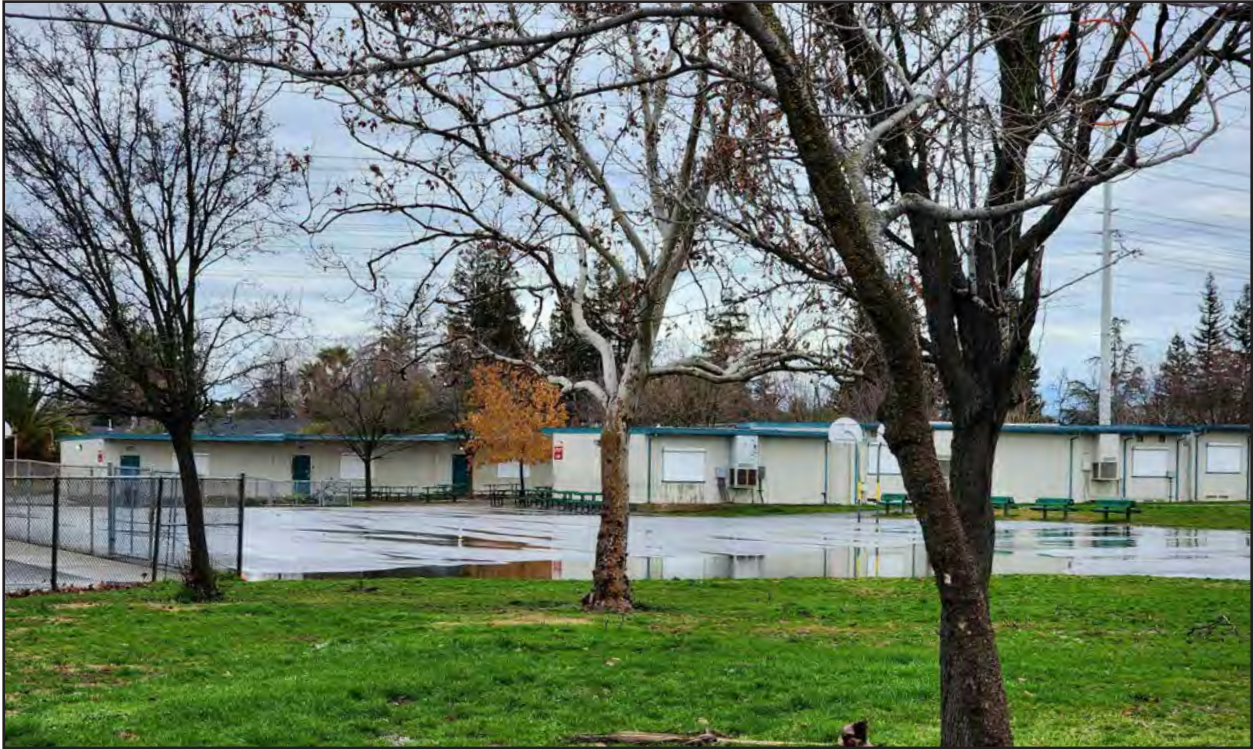
View of Nicholas Elementary School portables and hardcourts.
