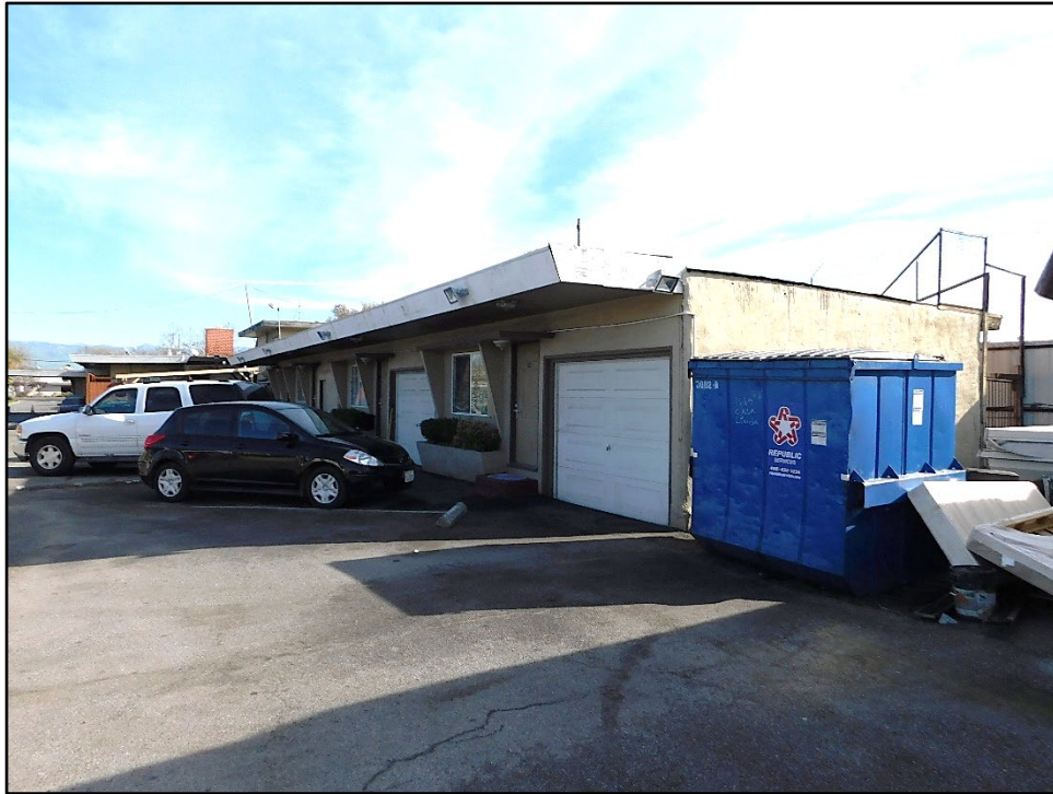
Photograph 7: Building B, camera facing east; January 14, 2022.
