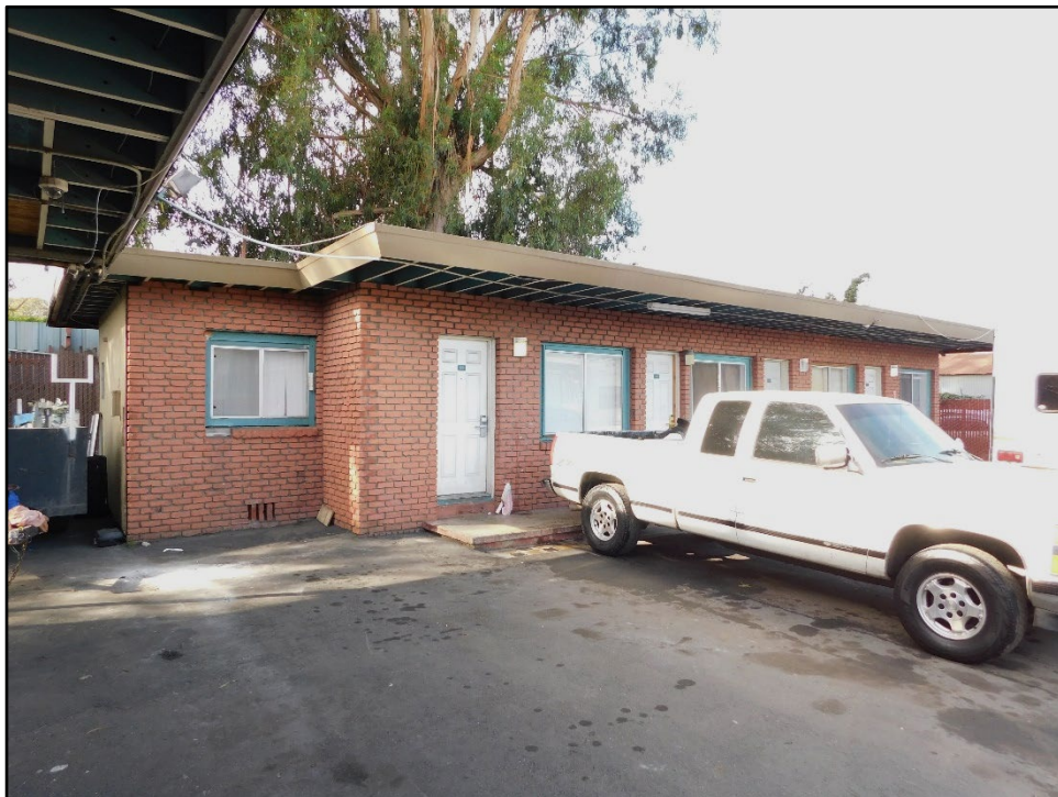
Photograph 14: Building F, camera facing west; January 14, 2022.
