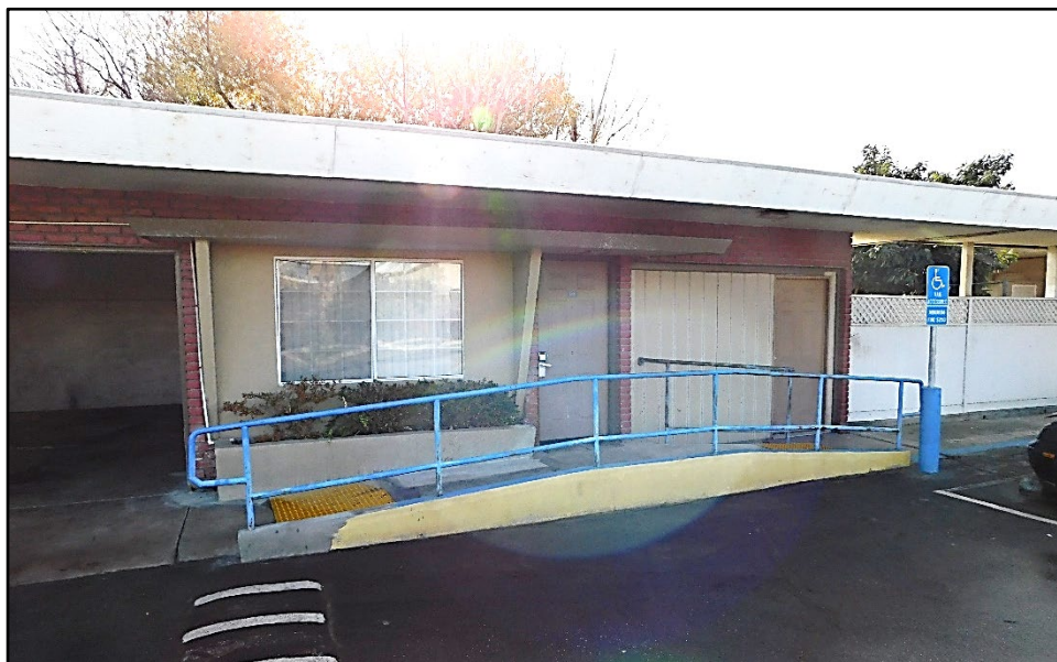
Photograph 10: Building C, camera facing southeast; January 14, 2022.
