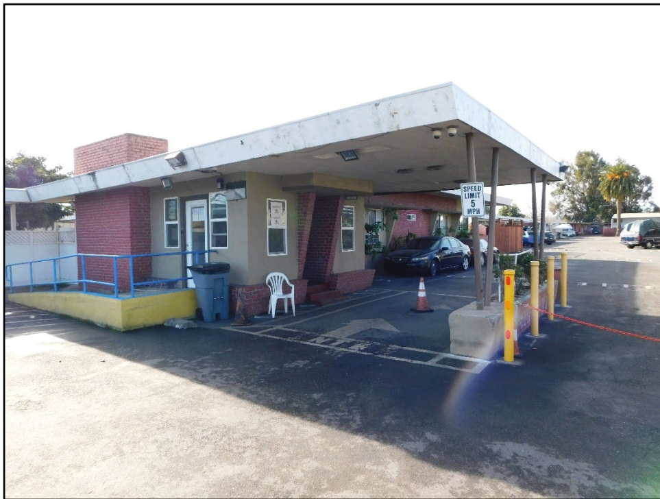
Photograph 4: Motel office, camera facing south; January 14, 2022.
