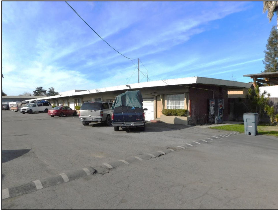
Photograph 11: Building D, camera facing west; January 14, 2022.
