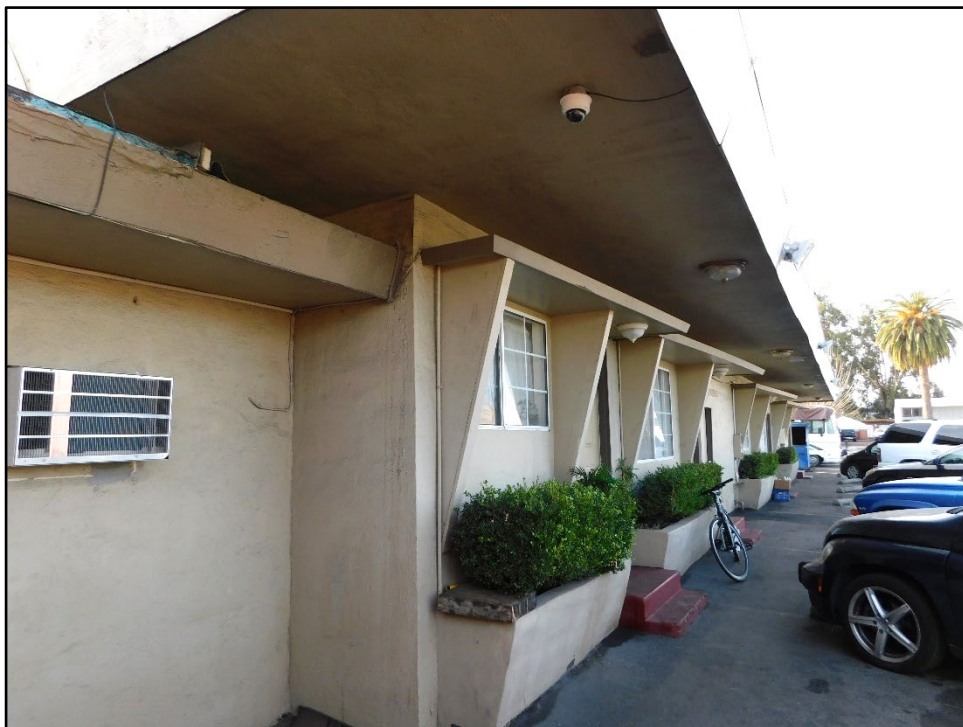
Photograph 8: Building B, camera facing south; January 14, 2022.
