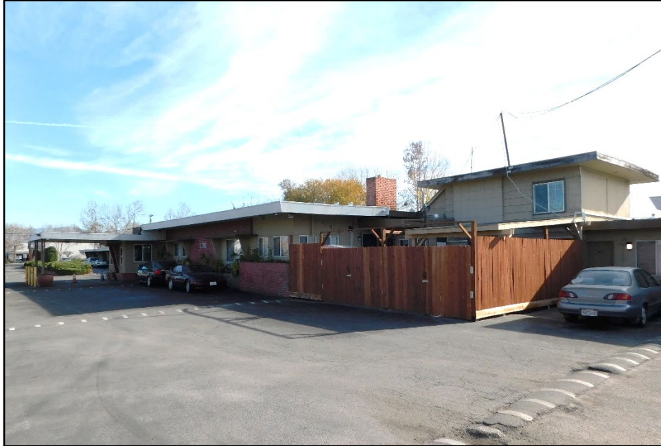
Photograph 3: Building A, camera facing east; January 14, 2022.
