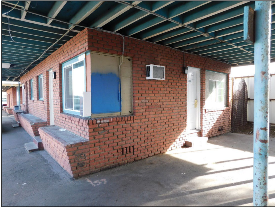
Photograph 13: Building E, camera facing east; January 14, 2022.
