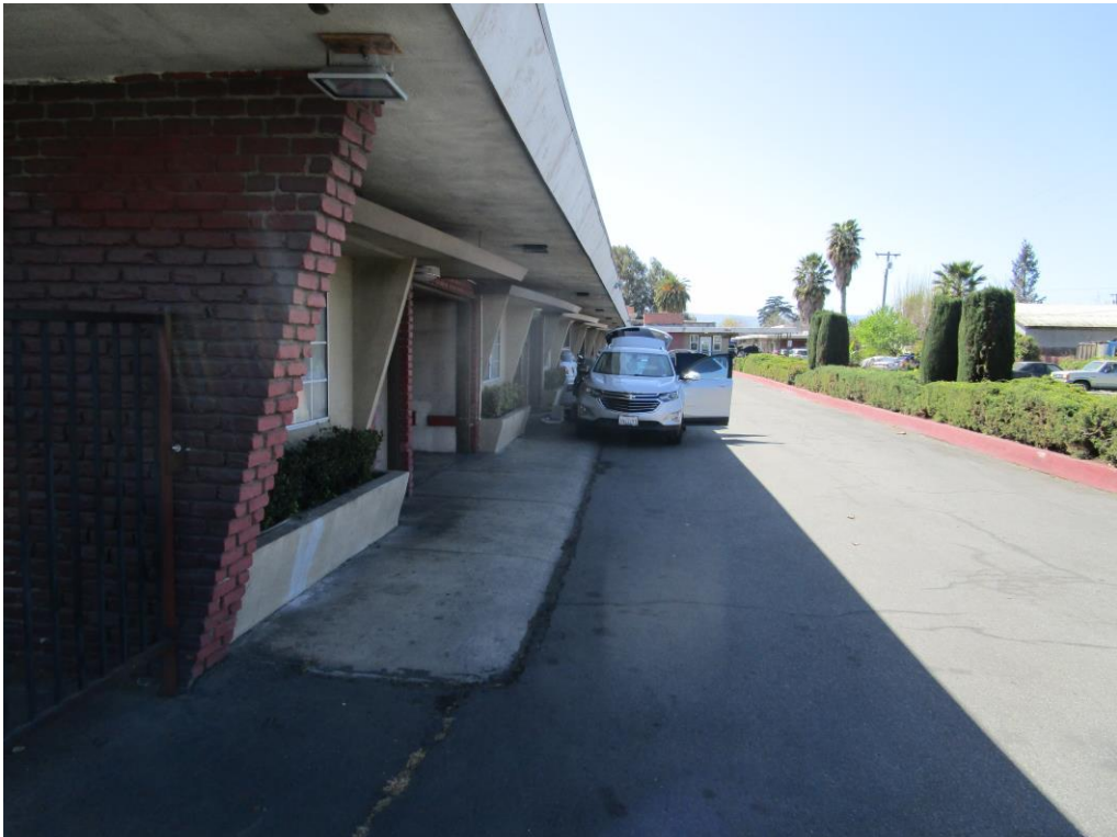
Photo 6: View of subject property from the east facing southeast.
