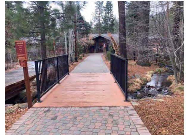
Bridge to NPOA Recreation Center
