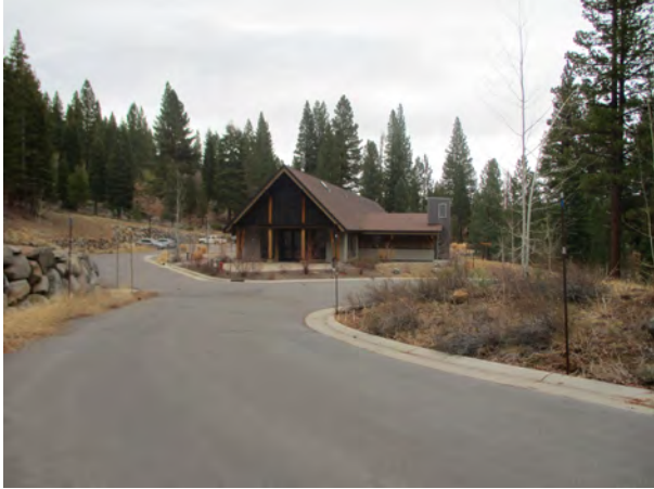
900 Northstar Drive - Southwest Elevation
