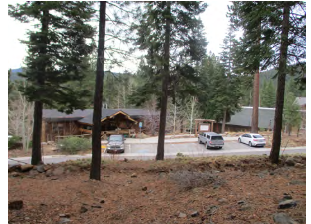
Trail View, 908 Northstar Drive - West Elevation
