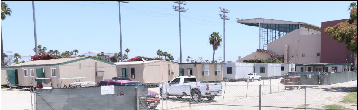
Modular buildings west of the Grandstand, view northeast (June 10, 2022).
