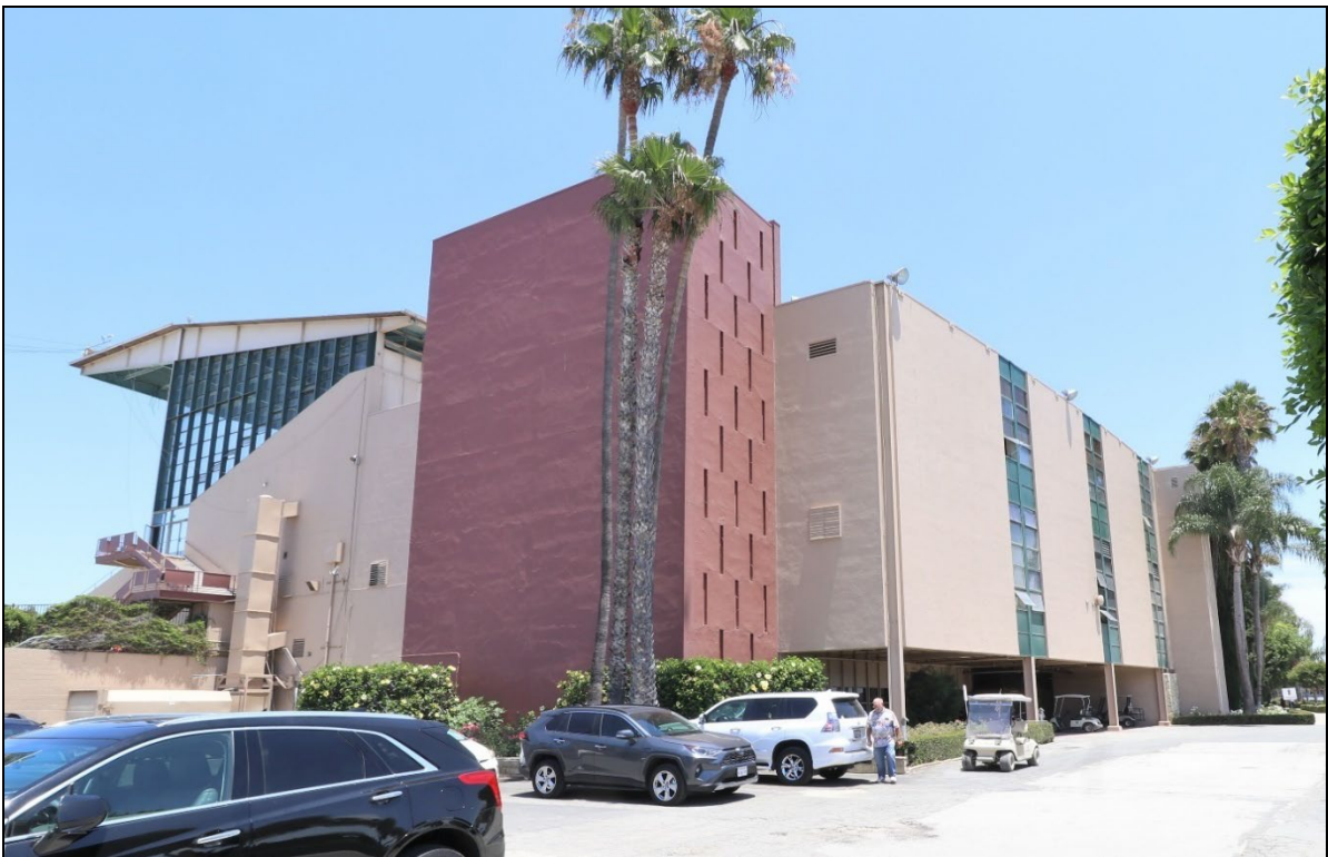
Grandstand, west and south elevations, view northeast (June 10, 2022).
