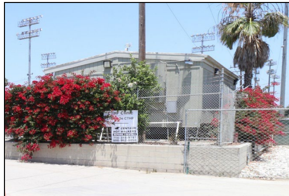
View northwest (June 10, 2022).
