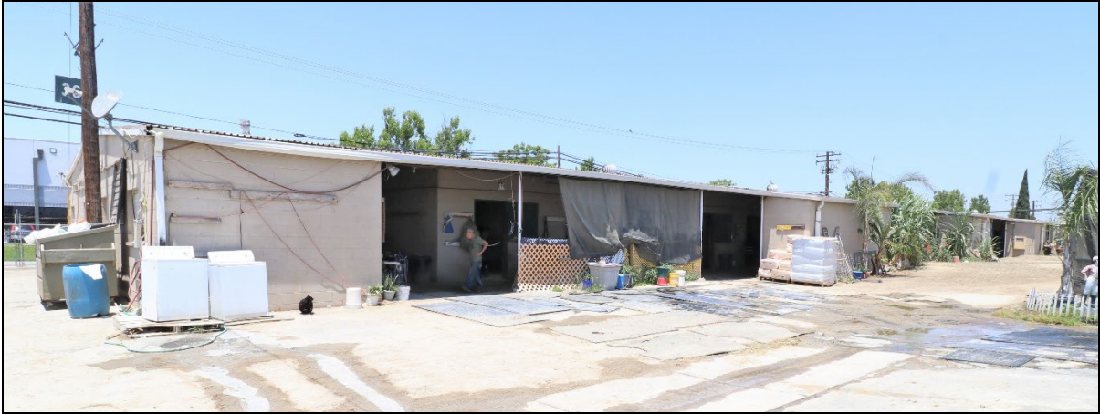
Barn. Typical historic-period barn. North and west elevations, view southeast (June 10, 2022).
