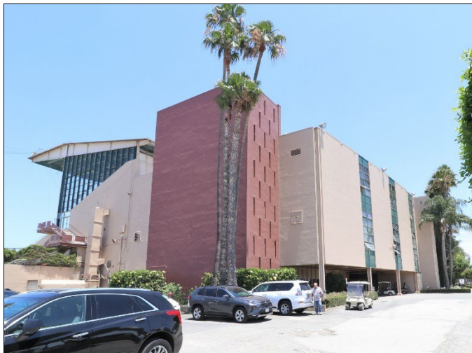
Grandstand, west and south elevations, view northeast (June 10, 2022).
