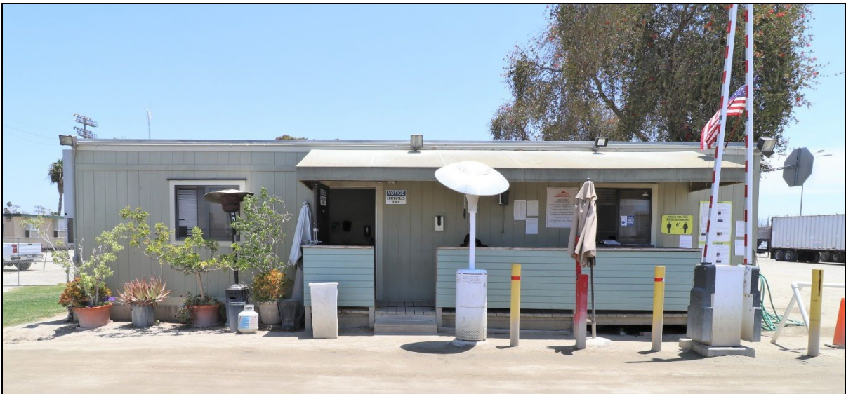
Check-in office, view to the east (June 10, 2022).
