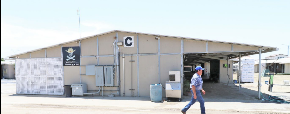
Typical modern barn. North elevation, view south (June 10, 2022).
