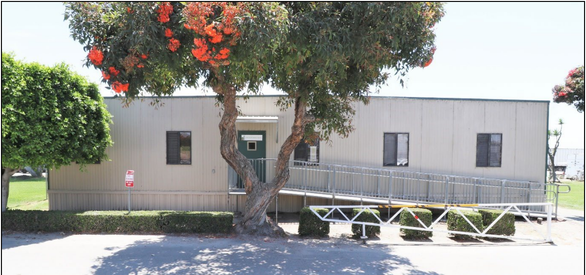
Modular building southwest of the Grandstand and north of the parking lot, view south (June 10, 2022).
