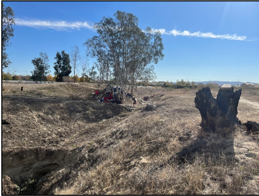
Figure 5-3. Overview of drainage channel in eastern portion of Project site, facing south
