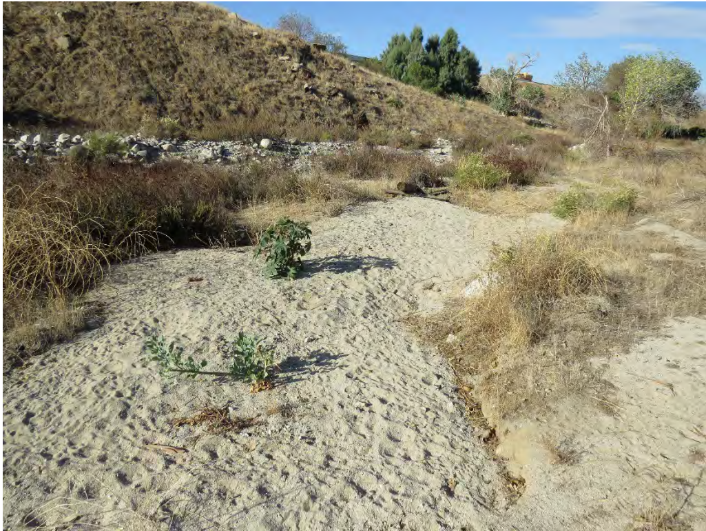
Photograph 12: Drainage 1 downstream of the culverts.
