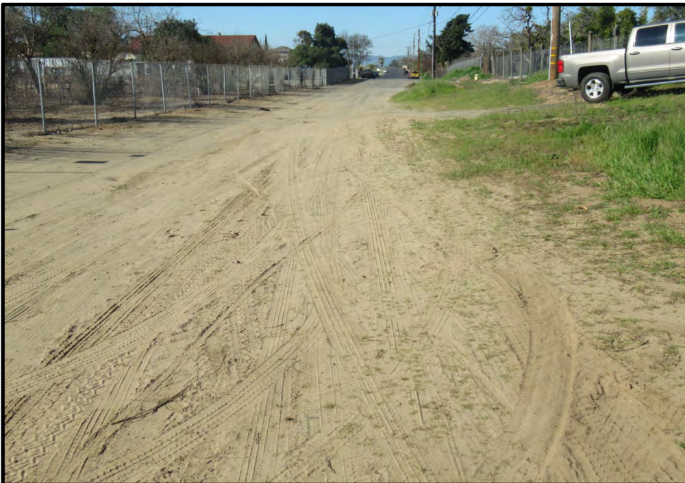
Hanson Lane, looking west from near the southeast corner of the site; 01/25/22. A sidewalk will be constructed along the north side of Hanson Lane for 320 feet to the west.
