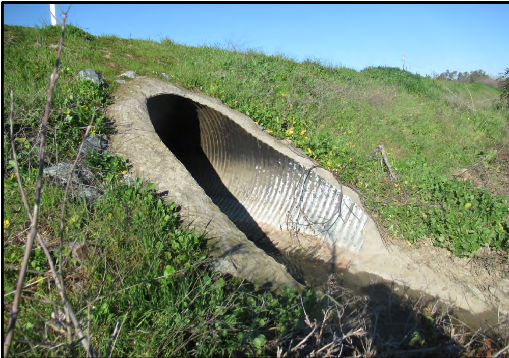
Close-up of the storm drain outfall structure, looking northwest; 01/25/22.
