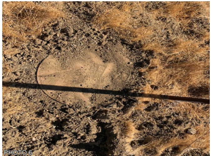
PHOTO 6 CENTRAL PORTION OF THE PROPERTY - SEWER MANHOLE
