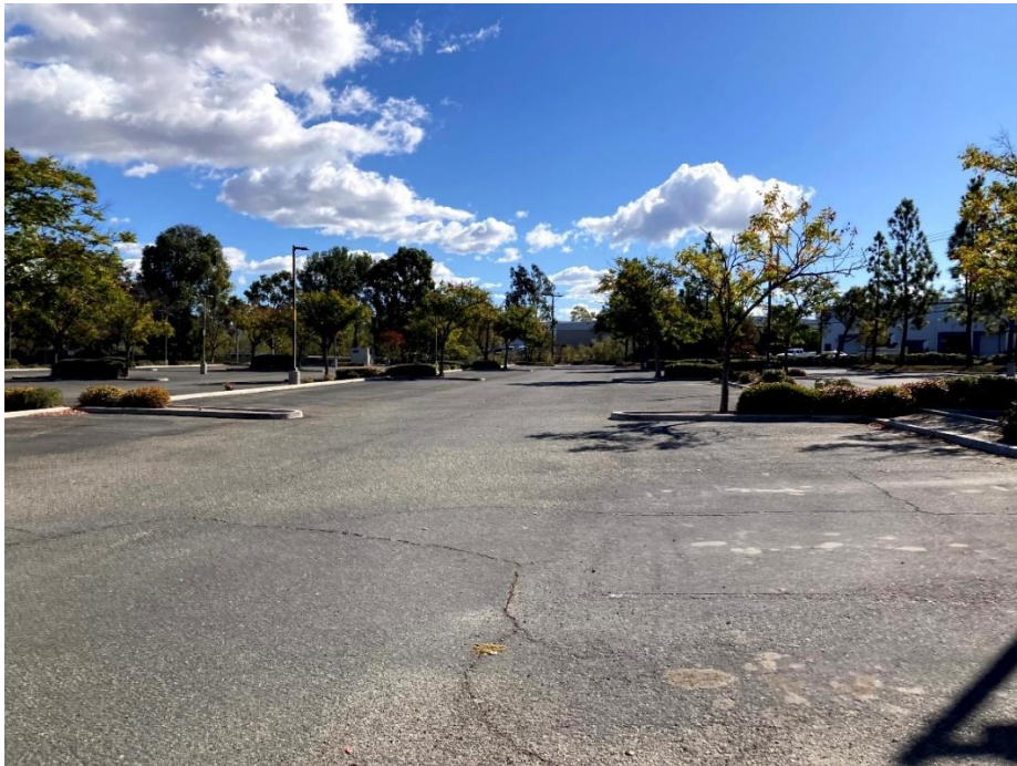
Figure 11. APE overview from western side looking east, November 3, 2022.
