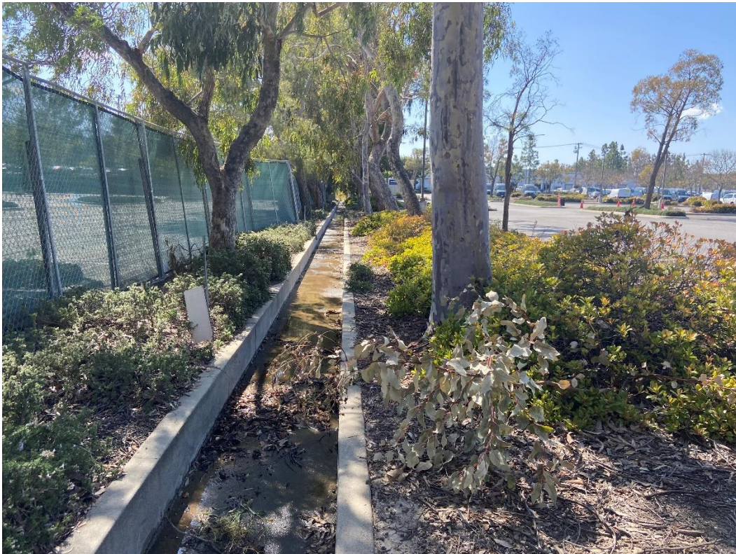
Photograph 2: Storm gutter along the eastern edge of the Property.
