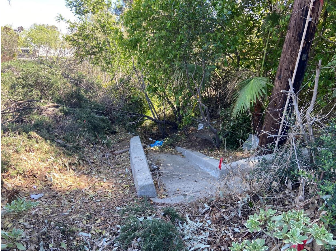
Photograph 11: Stormwater drainage are in the southeast corner.
