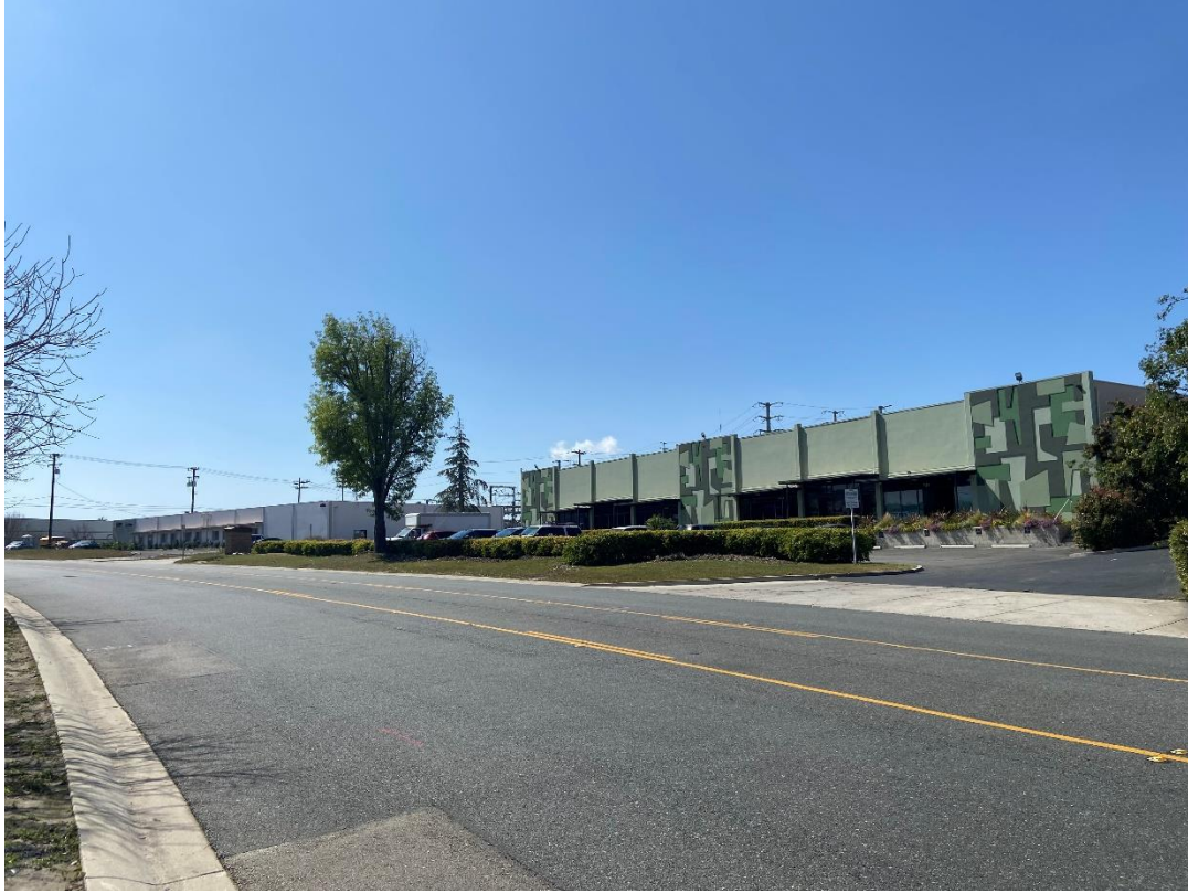
Photograph 5: Western adjoining properties.
