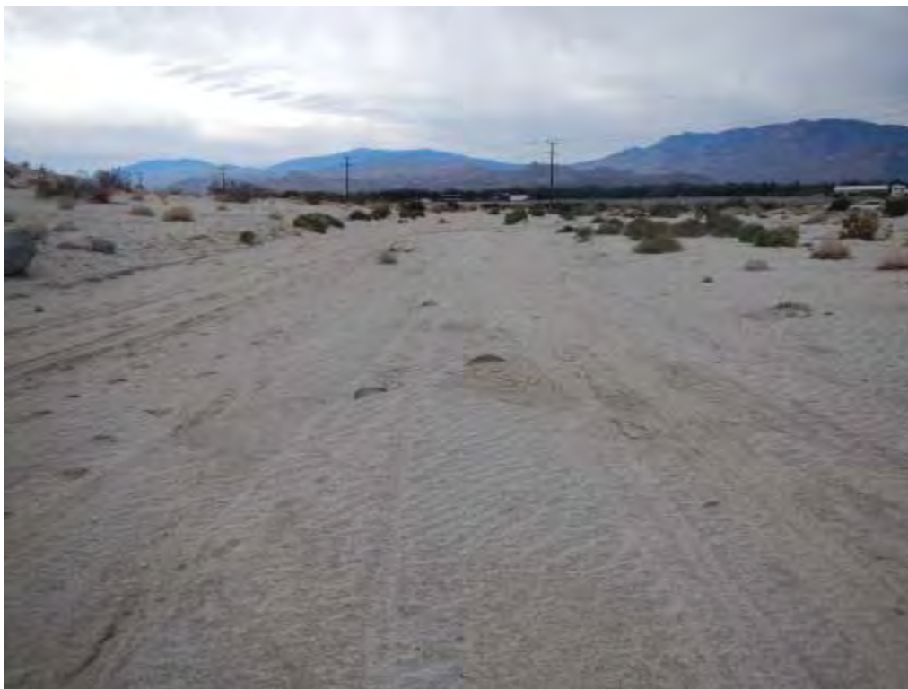
Photograph 10 – Looking south (downstream) at the wide low flow channel and active floodplain within Reach 3.
