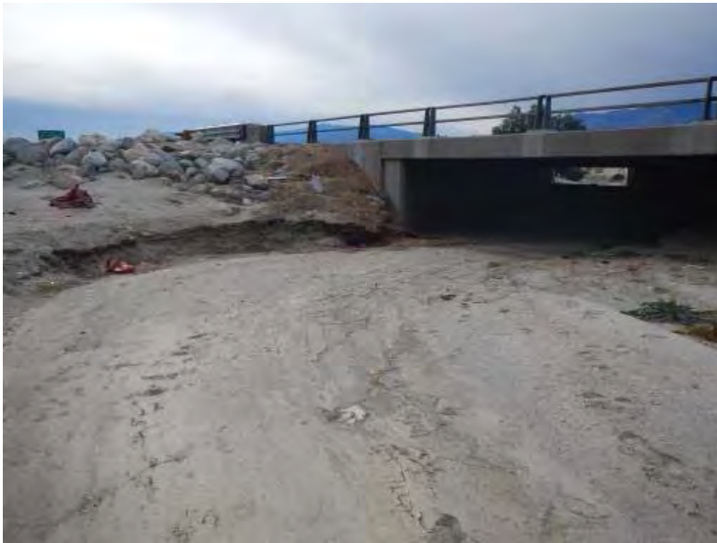
Photograph 7 – Looking south (downstream) at the Reach 2 I-10 crossing.
