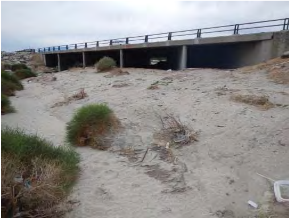
Photograph 1 – Looking south (downstream) at the Reach 1 I-10 bridge crossing.
