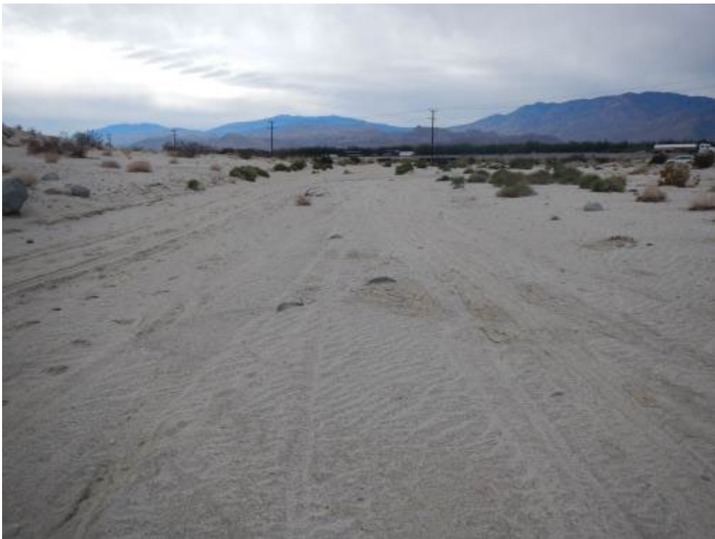
Photograph 10 – Looking south (downstream) at the wide low flow channel and active floodplain within Reach 3.
