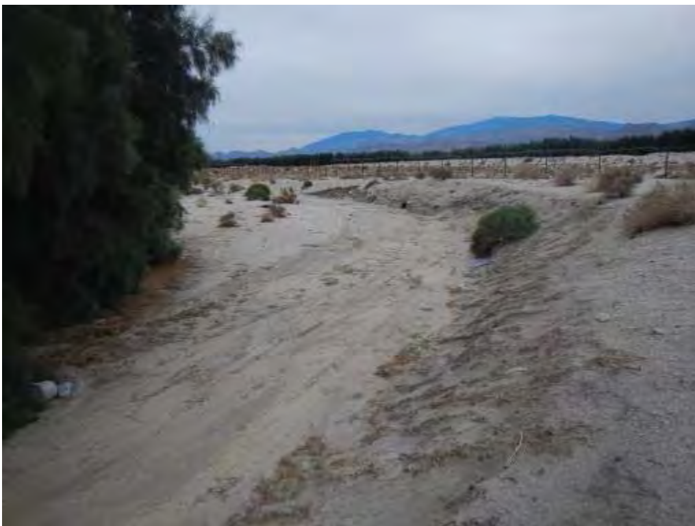
Photograph 24 – Looking south (downstream) immediately downstream of the Reach 2 I-10 crossing.
