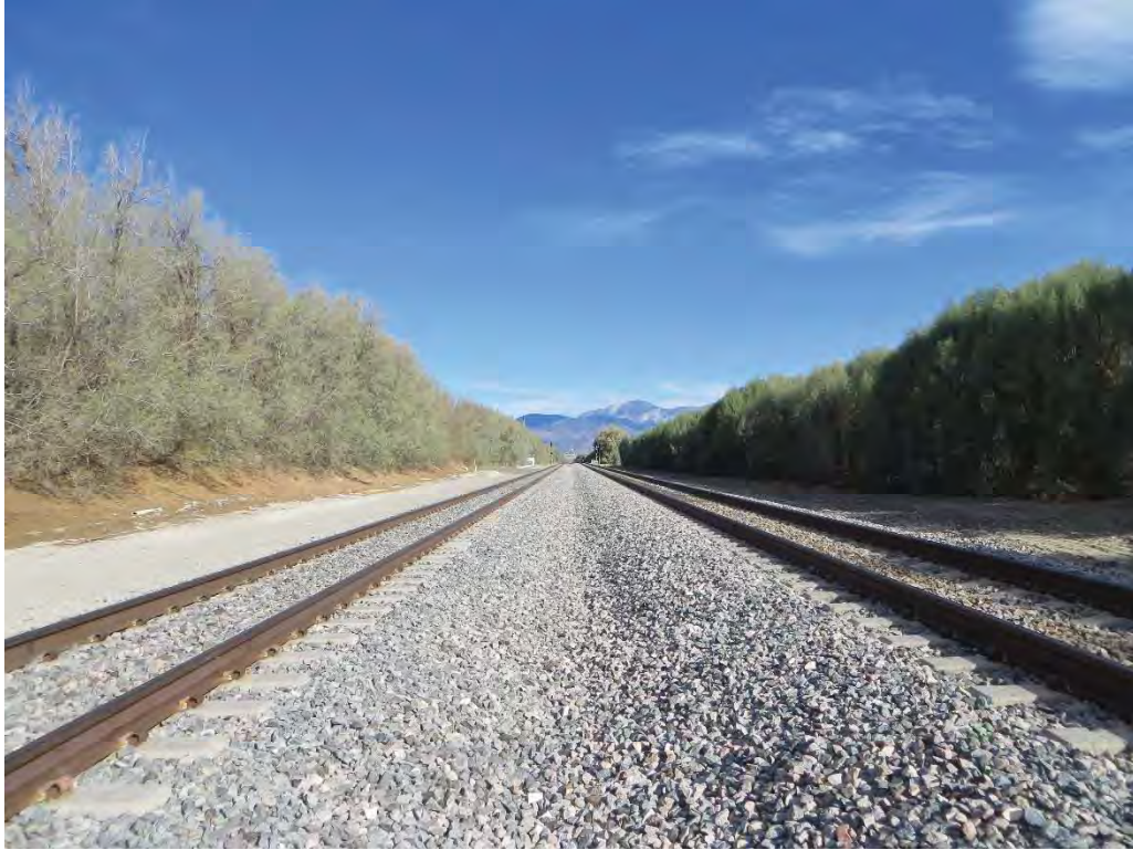
Photograph 5: Facing west from the center of the railroad tracks. Tamarisk windrows are located both to the north and south. The tracks and these windrows restrict aeolian sand transport between areas to the north and south.
