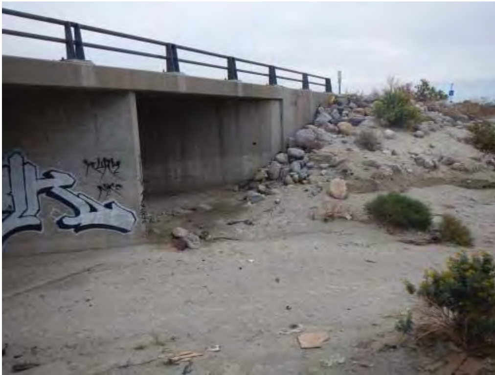
Photograph 15 – Looking northeast at the southern side of the Reach 1 I-10 crossing.
