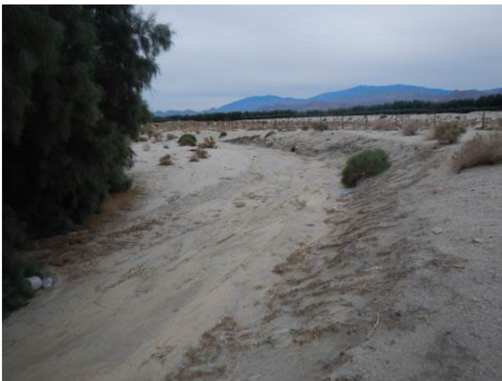
Photograph 24 – Looking south (downstream) immediately downstream of the Reach 2 I-10 crossing.
