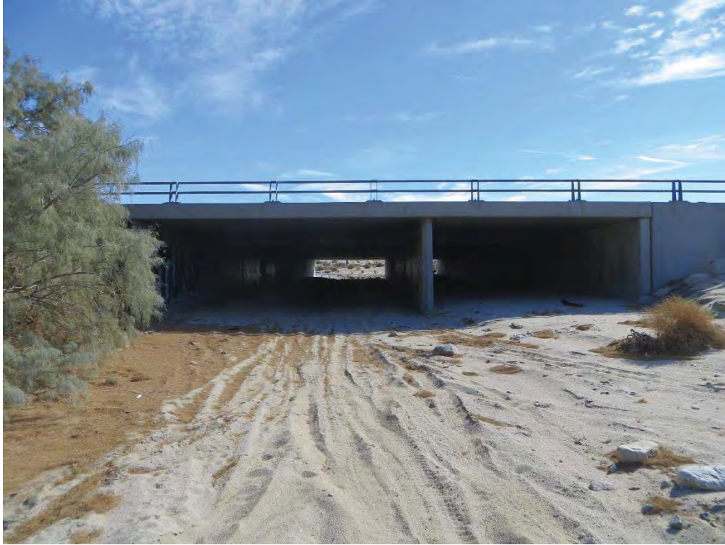
Photograph 9: Facing north. This crossing allows movement of wildlife, water, and sand under Interstate 10. However, because of the windrows and railroad tracks, water is currently restricted once it enters the area between the interstate and railroad tracks.
