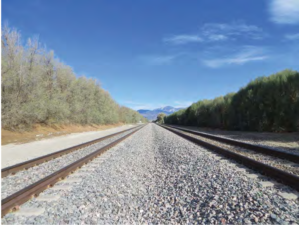
Photograph 5: Facing west from the center of the railroad tracks. Tamarisk windrows are located both to the north and south. The tracks and these windrows restrict aeolian sand transport between areas to the north and south.
