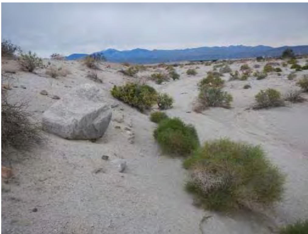
Photograph 18 – Looking northwest (upstream) along the southern border of Reach 1. The artificial berm confines Morongo Wash to a specific area.
