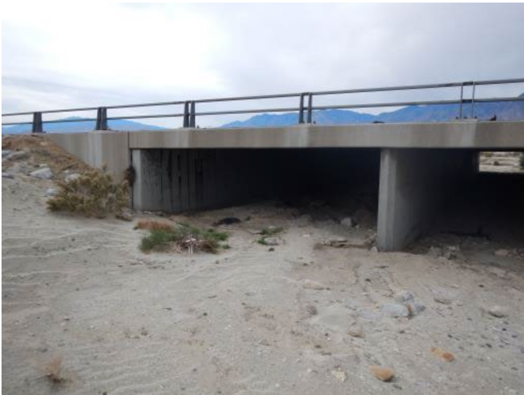
Photograph 14 – Looking south (downstream) at the Reach 3 I-10 crossing.
