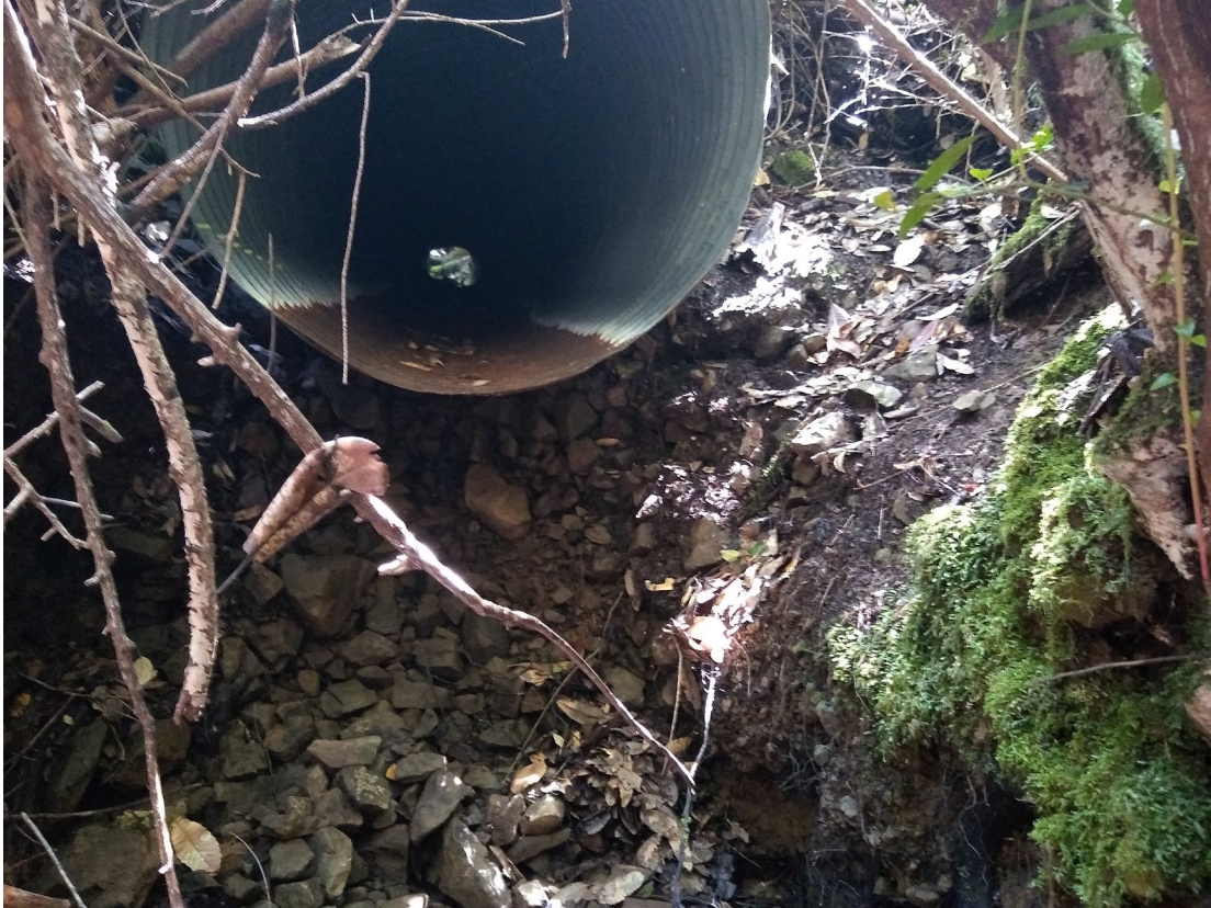
Figure 4. Outlet of existing culvert at proposed POD location.
