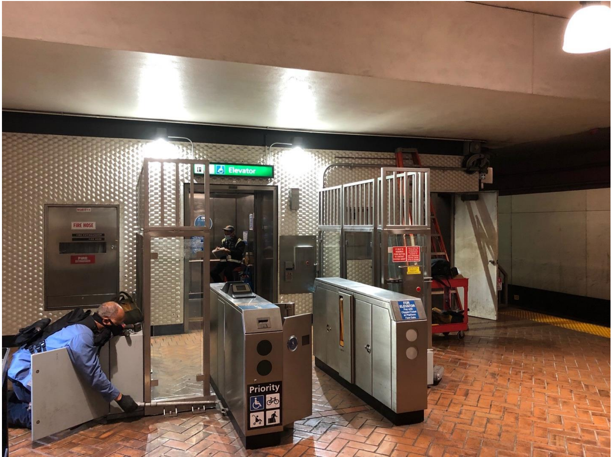
Photo of Fare Gate and Enclosure at Elevator to Street
