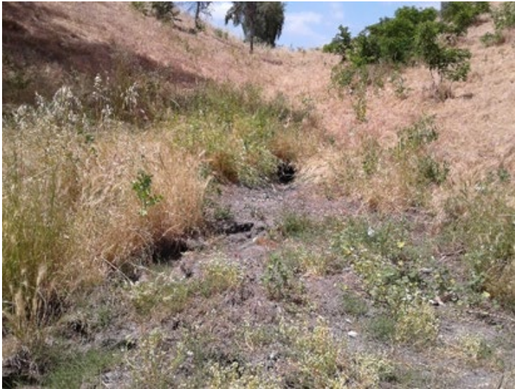
Figure 2-10 Highway Stormwater Conveyance at the Northern Point of Potential Wetland Location-01
