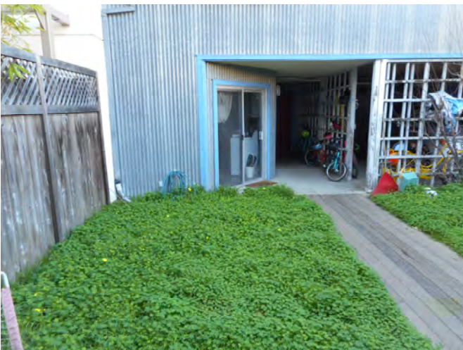
Photo 5: View of garage/laundry room from yard area looking west.
