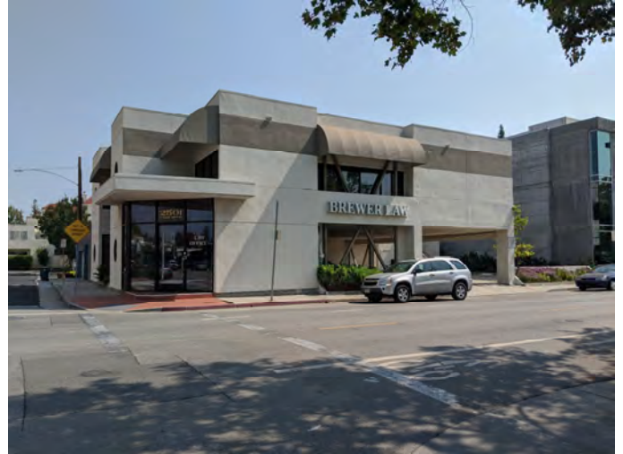
Photo 2: Front of site building looking north across Park Boulevard.
