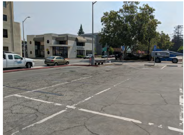
Photo 4: Site building in photo background from public parking lot looking east.
