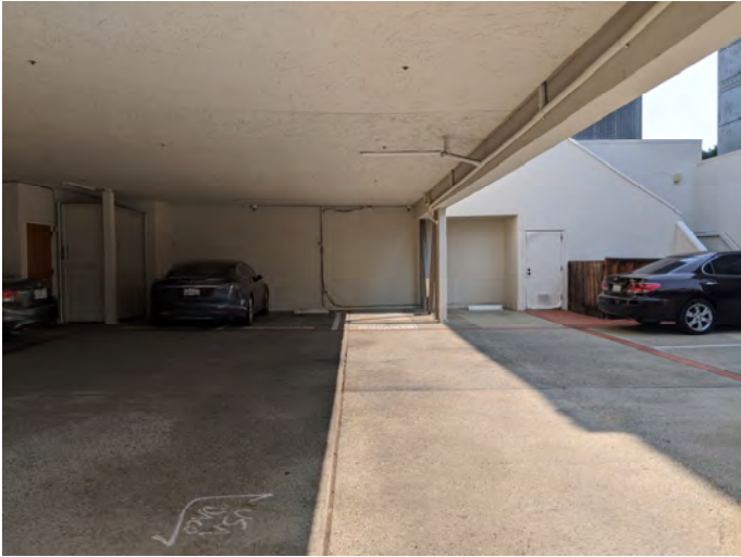
Photo 7: Covered portion of site parking lot looking northeast.
