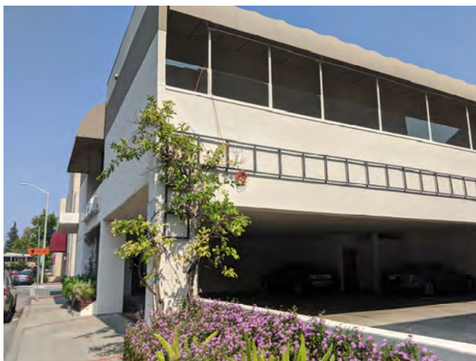
Photo 5: Site building and covered parking from Park Boulevard sidewalk.
