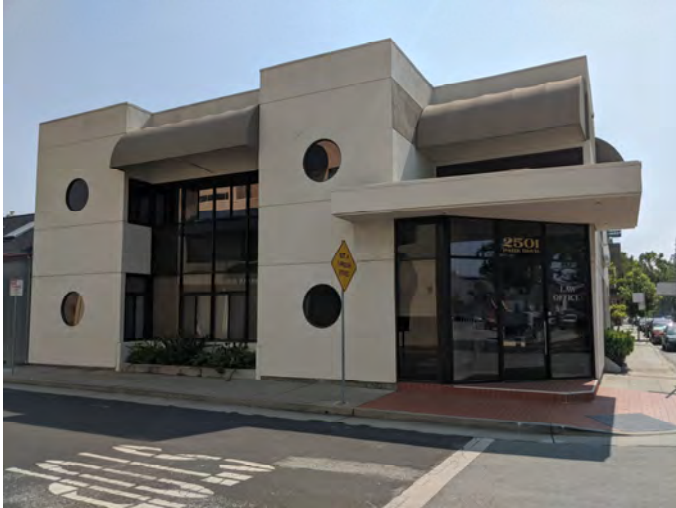
Photo 1: Front of site building looking east across Sherman Avenue.
