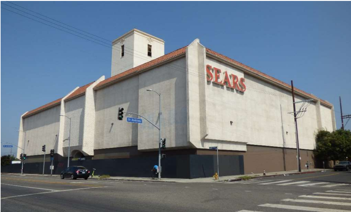
South and east façades, view facing northwest.
