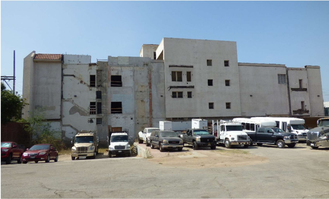
North (rear) façade, view facing southwest.
