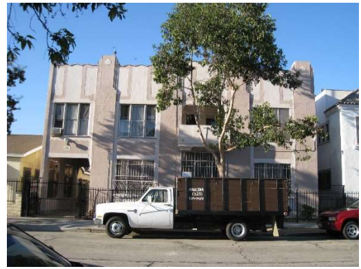
5623 Virginia Ave, 2019. Source: Architectural Resources Group.
