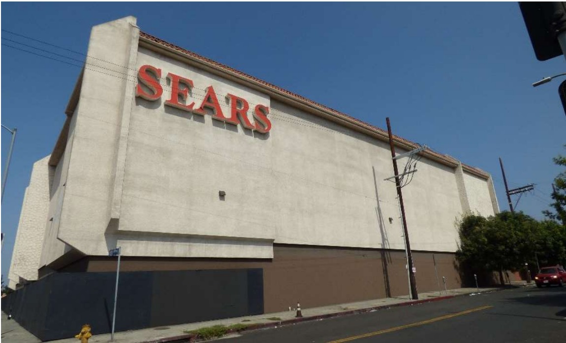
East façade, view facing northwest.
