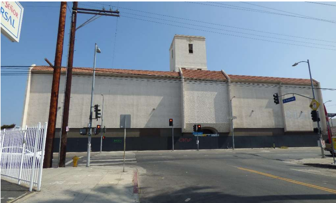
South (primary) façade, view facing northeast.
