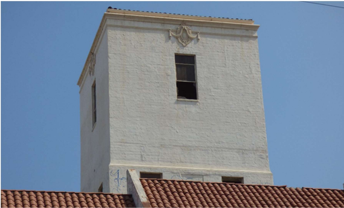
Tower detail, view facing northeast.
