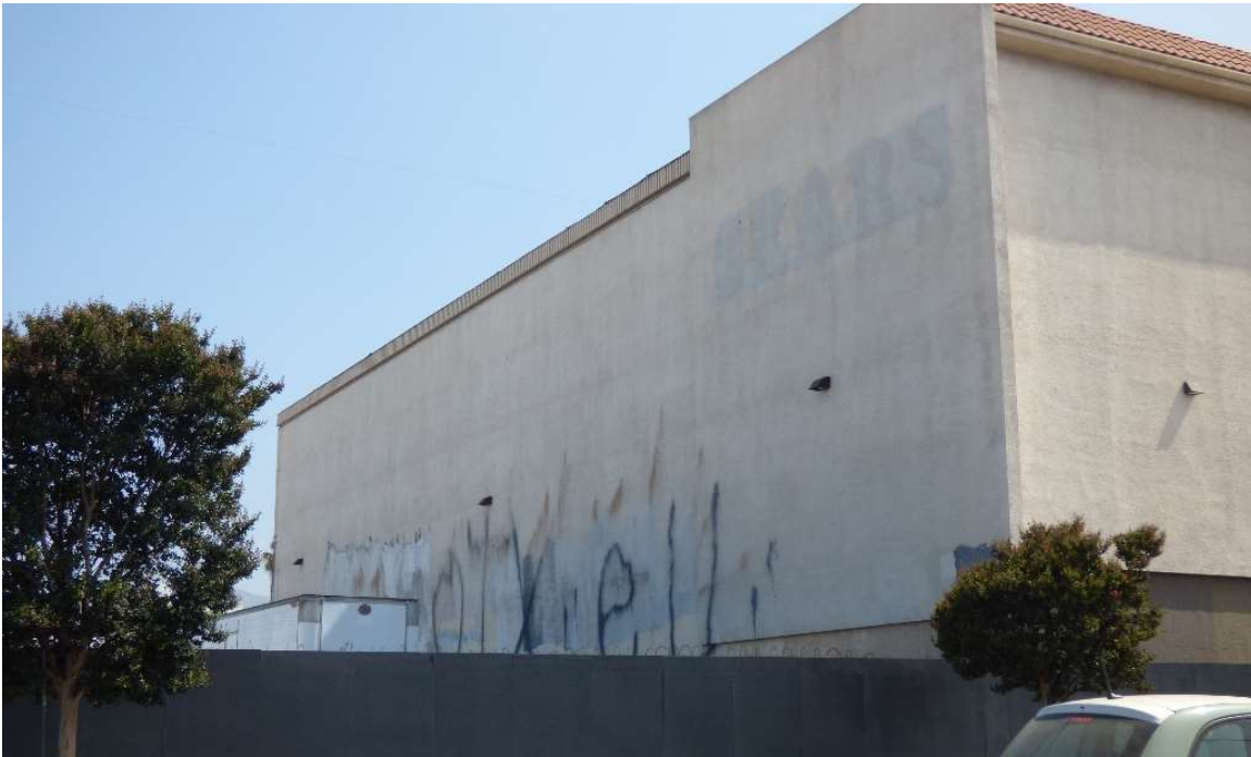
West façade, view facing northeast.
