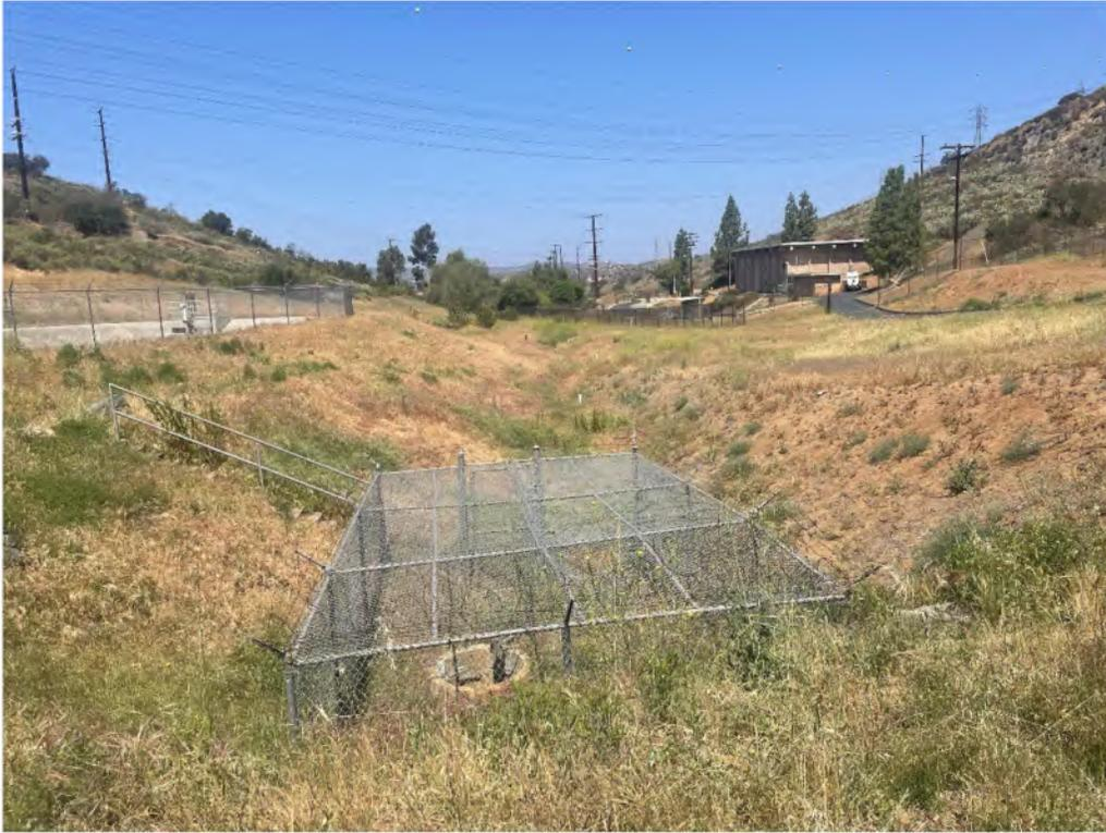
**Photo 13.** View facing northwest along swale and dam weir structure at base of dam. Sump is visible in foreground, with pump stations visible in background at right.
