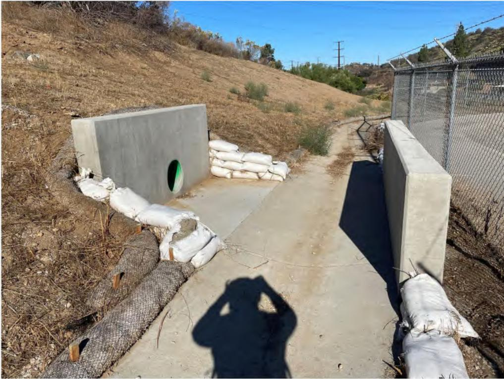
**Photo 7.** View facing northwest along concrete-lined channel CC-3 and culvert outlet connected to RWQCB-jurisdictional earthen-lined channel EC-1. This concrete channel flows into a non-jurisdictional swale.
