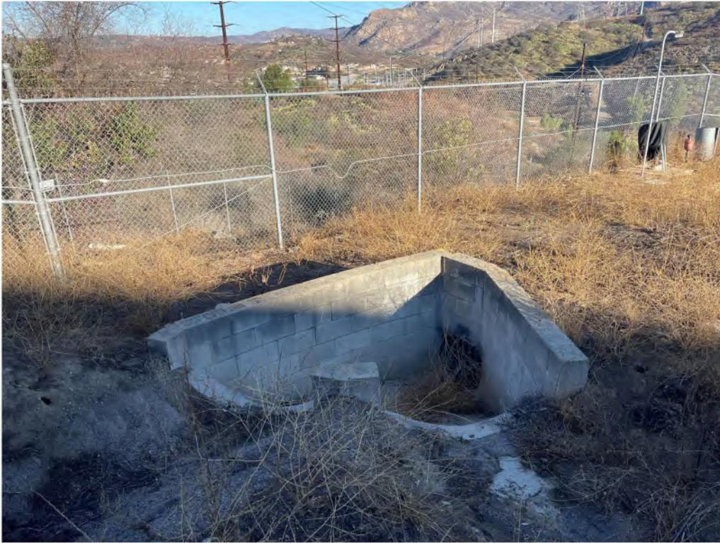
**Photo 3.** View facing northwest of primary culvert inlet draining water treatment plant stormwater runoff, with two RWQCB-jurisdictional channels feeding into it (features AC-1 and BD-5). Culvert is located in northwestern corner of water treatment plant.
