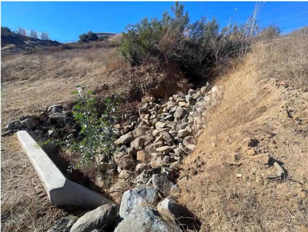
**Photo 6.** View facing south at downstream portion of RWQCB-jurisdictional earthen-lined channel EC-1. Rip-rap, artificial banks and a culvert inlet is visible in foreground.
