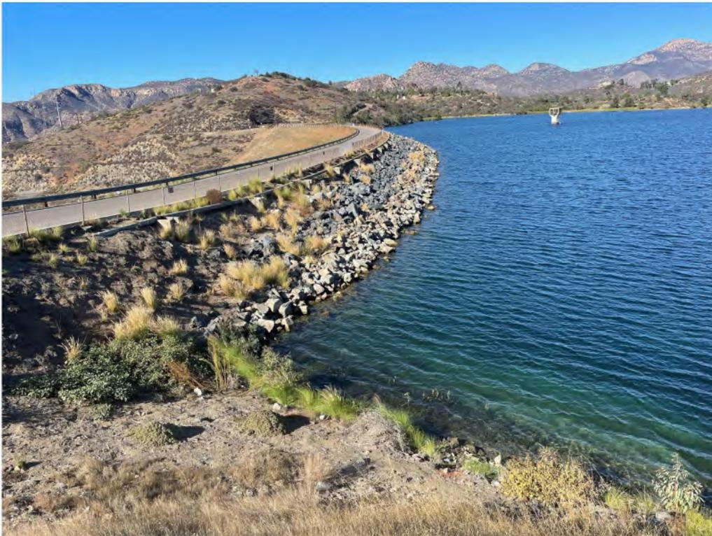
**Photo 26.** View facing north along Chet Harritt Dam from its southern abutment. An OHWM is visible about halfway up the rip-rap slope at center.
