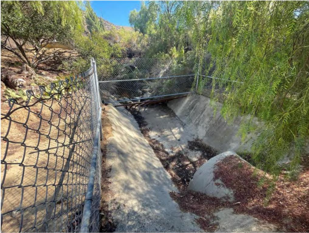
**Photo 19.** View facing east/upstream along non-wetland waters feature NWW-D-4, which is a concrete-lined channel ultimately connected to the dam spillway. This channel conveys flows along this feature offsite, where it appears to continue through a series of culverts and channels to Lindo Lake and/or the San Diego River.
