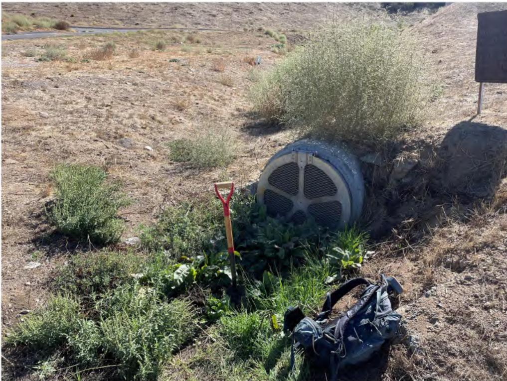
**Photo 10.** View facing east along non-jurisdictional swale, culvert outlet of water treatment plant detention basin and Wetland Sample Point UP-1. Although the area supported moist soils and herbaceous vegetation, no wetland indicators were observed.
