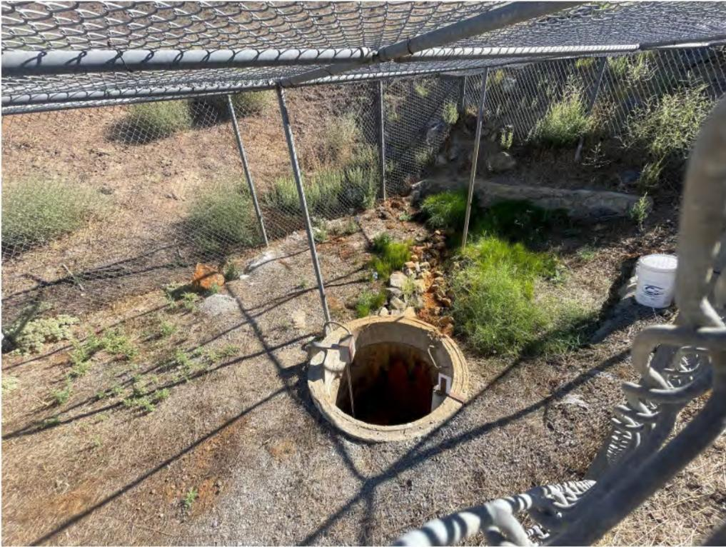
**Photo 9.** View facing east from within caged area of feature NWW-DS-1. Seepage from the earthen Chet Harritt Dam is consolidated and flows out of walled area in background into the circular drain in foreground where a weir is located to observe and measure the flow. This seepage is then pumped back to Lake Jennings. This short channel is considered jurisdictional to USACE, RWQCB and CDFW.
