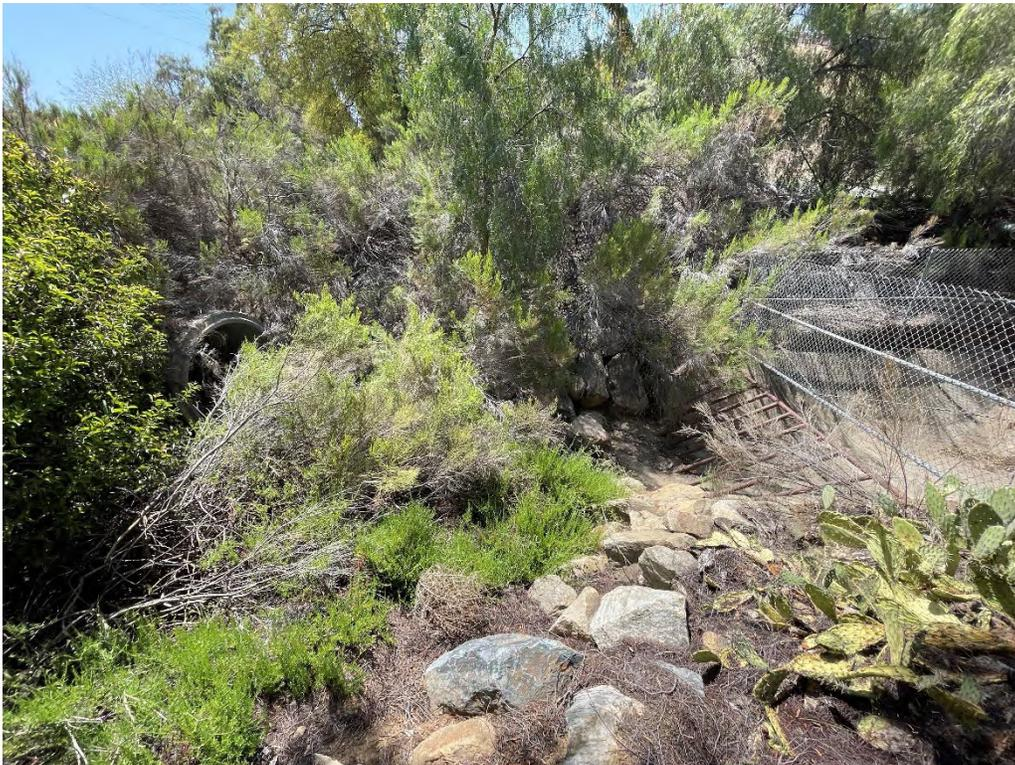
**Photo 14.** View facing south of culvert and debris guard near western boundary of study area. These culverts convey flow outside of the study area.
