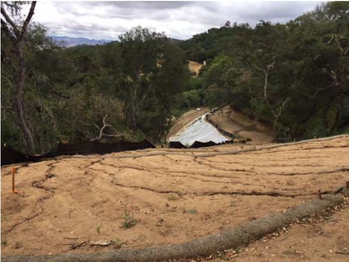
Figure 8. Erosion is occurring on steep upper section of road near the existing homesite. Refer to SWPPP that is being prepared to address erosion and sedimentation control issues.
