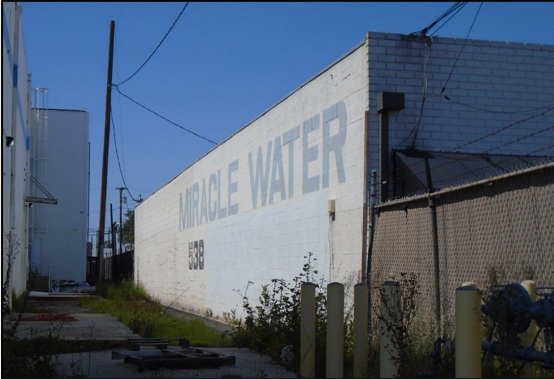
Figure 22. Building 3 (16835-16839 South Normandie Ave., APN 6106-030-015), south elevation, view northwest
