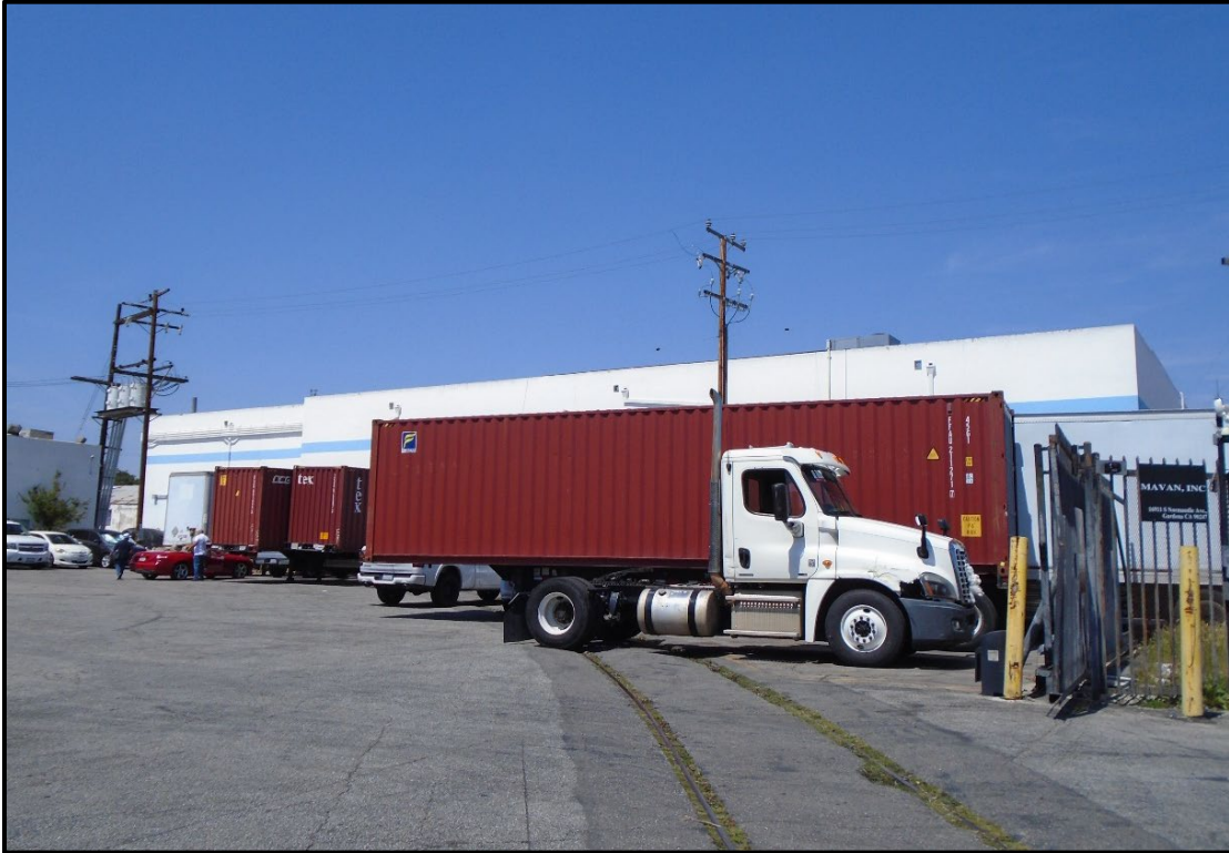
Figure 30. Building 4 eastern addition (16907 South Normandie Ave., APN 6106-030-017), south elevation, view northwest
