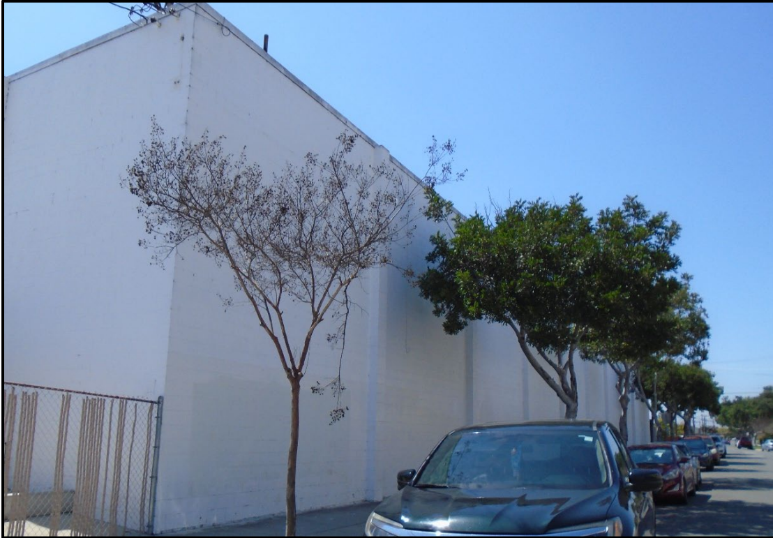
Figure 14. Building 1 (16829 South Normandie Ave., APN 6106-030-011), north elevation, view southwest
