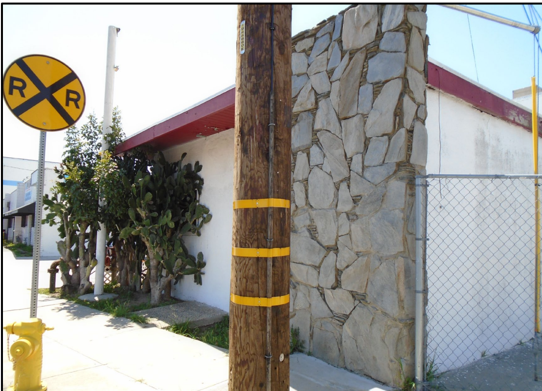
Figure 17. Building 2 (16829-16831 South Normandie Ave., APN 6106-030-011), east elevation, view southwest
