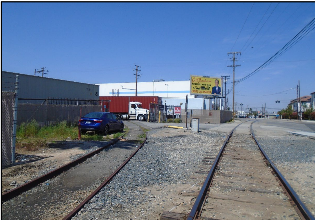
Figure 39. Railroad tracks on Normandie Avenue, with spur line entering the subject parcel, view north
