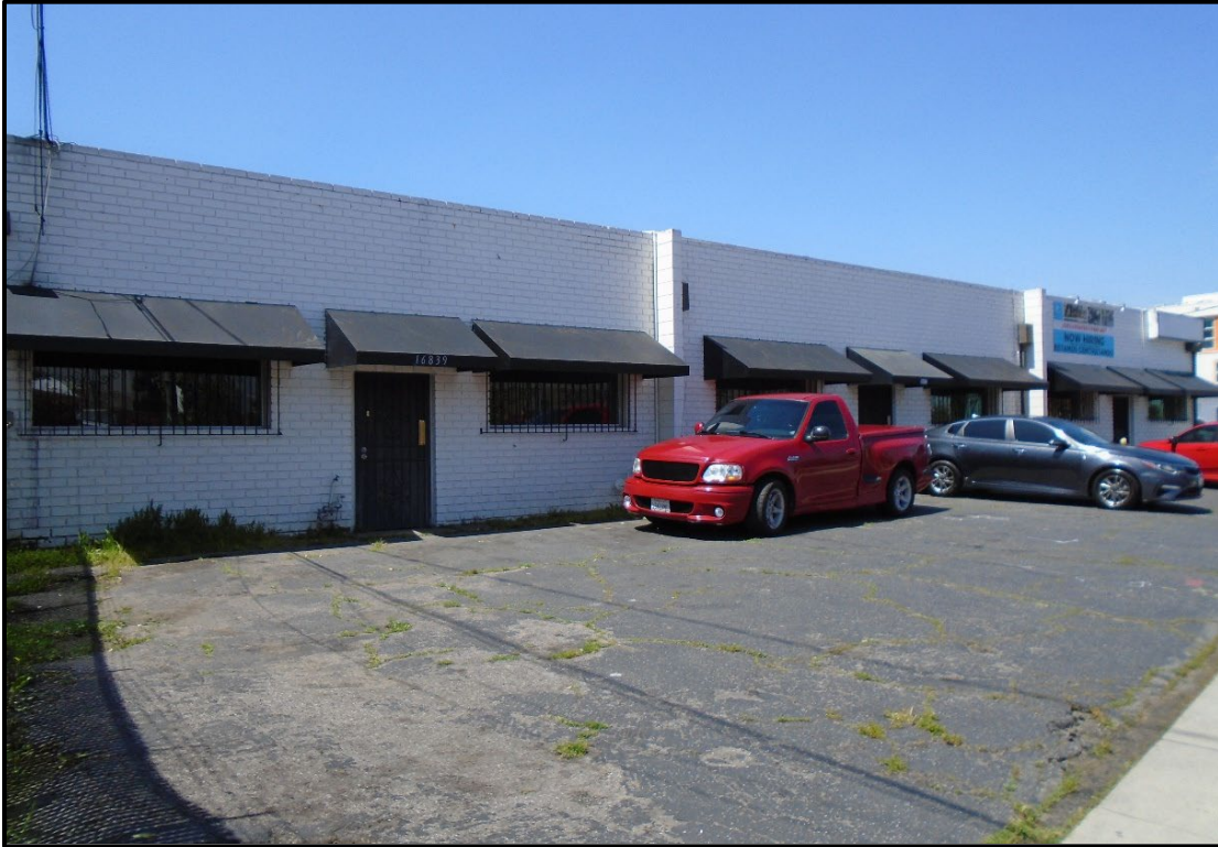
Figure 20. Building 3 (16835-16839 South Normandie Ave., APN 6106-030-015), east elevation, view northwest
