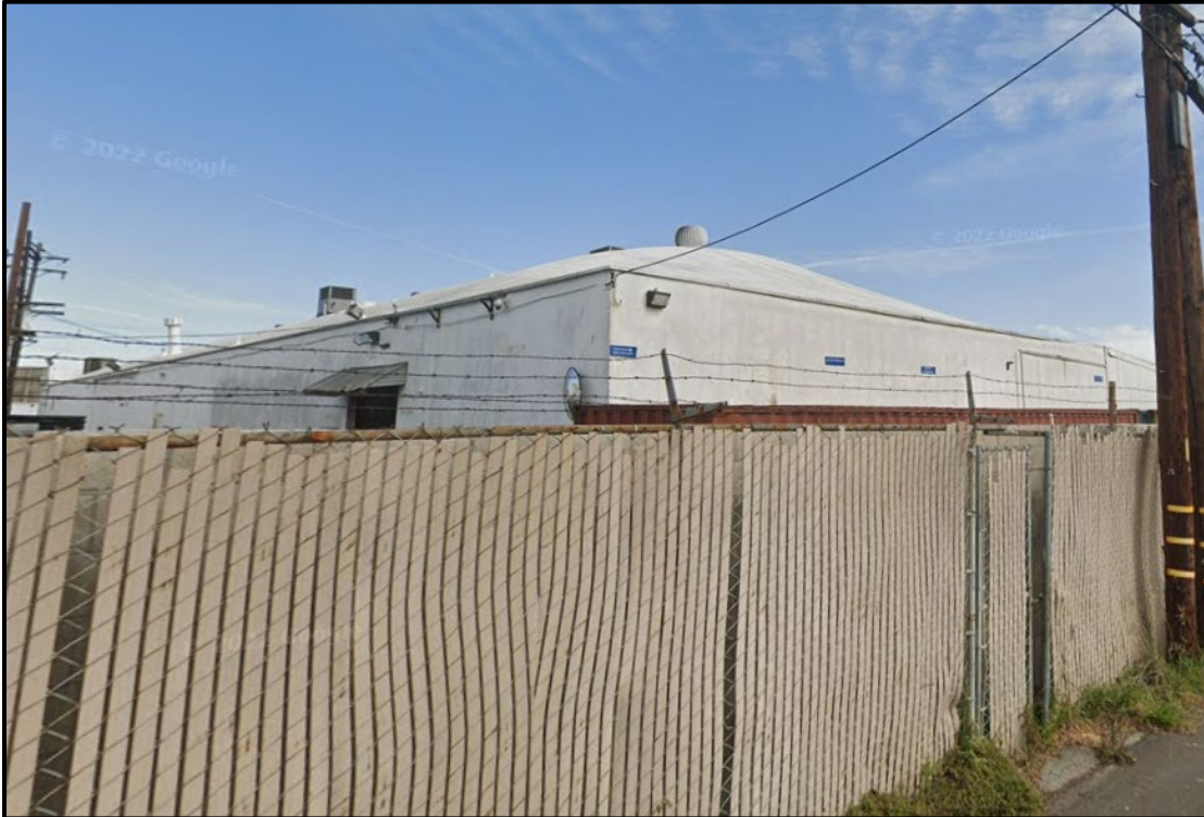
Figure 34. Building 5 (16911 South Normandie Ave., APN 6106-030-017), partial north and west elevations, view southeast
