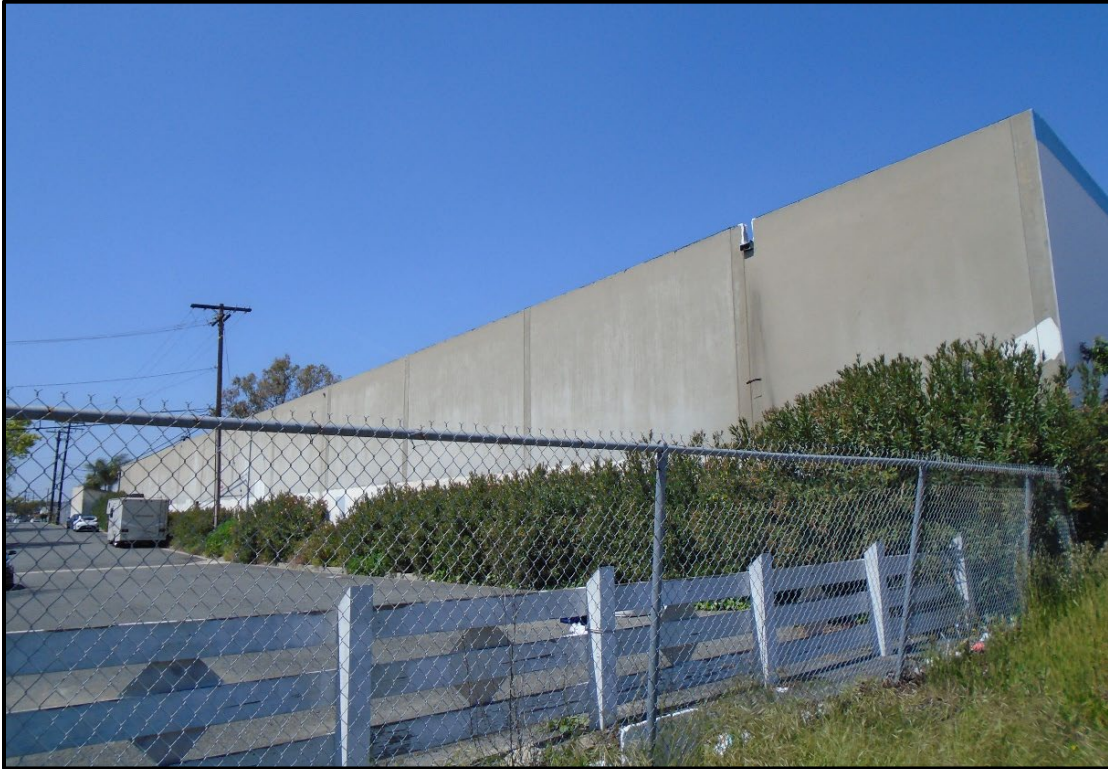
Figure 38. Building 6 (16911 South Normandie Ave., APN 6106-030-017), south elevation, view northwest
