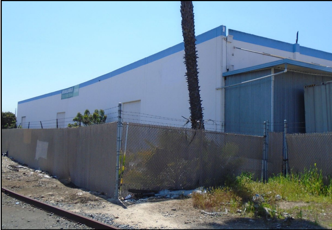
Figure 36. Building 6 (16911 South Normandie Ave., APN 6106-030-017), east elevation, view southwest
