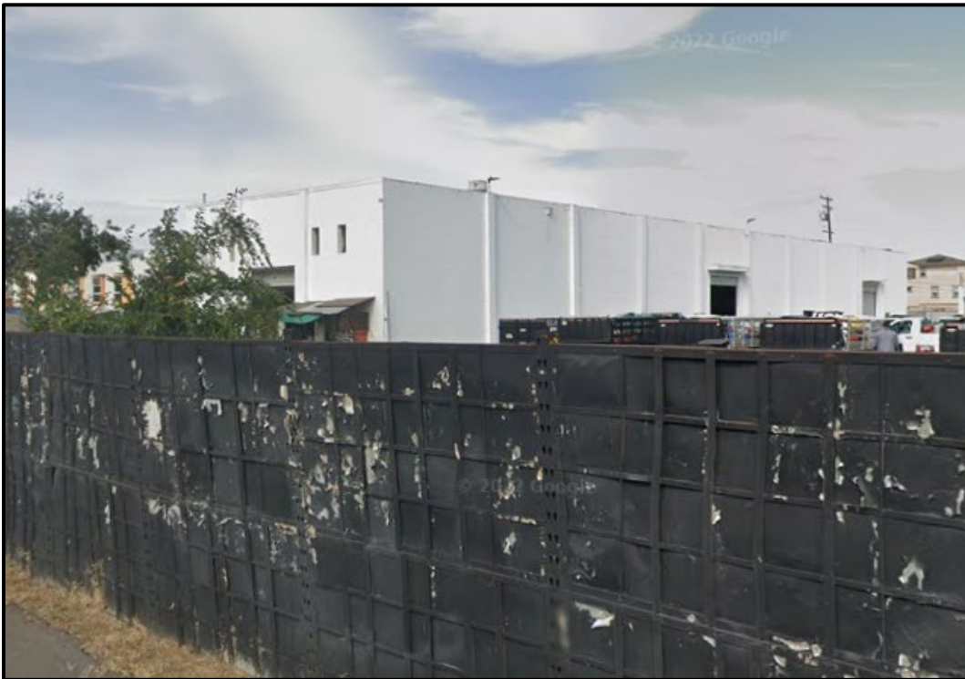
Figure 13. Building 1 (16829 South Normandie Ave., APN 6106-030-011), south and west elevations, view northeast
