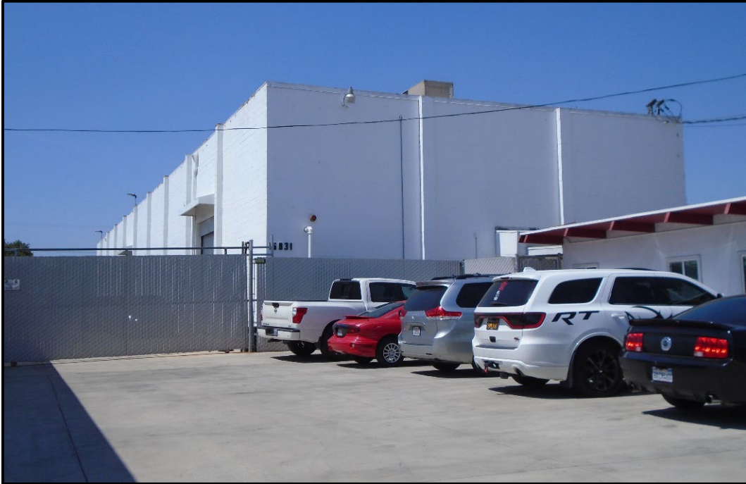
Figure 12. Building 1 (16829 South Normandie Avenue, APN 6106-030-011), south and east elevations, view northwest
