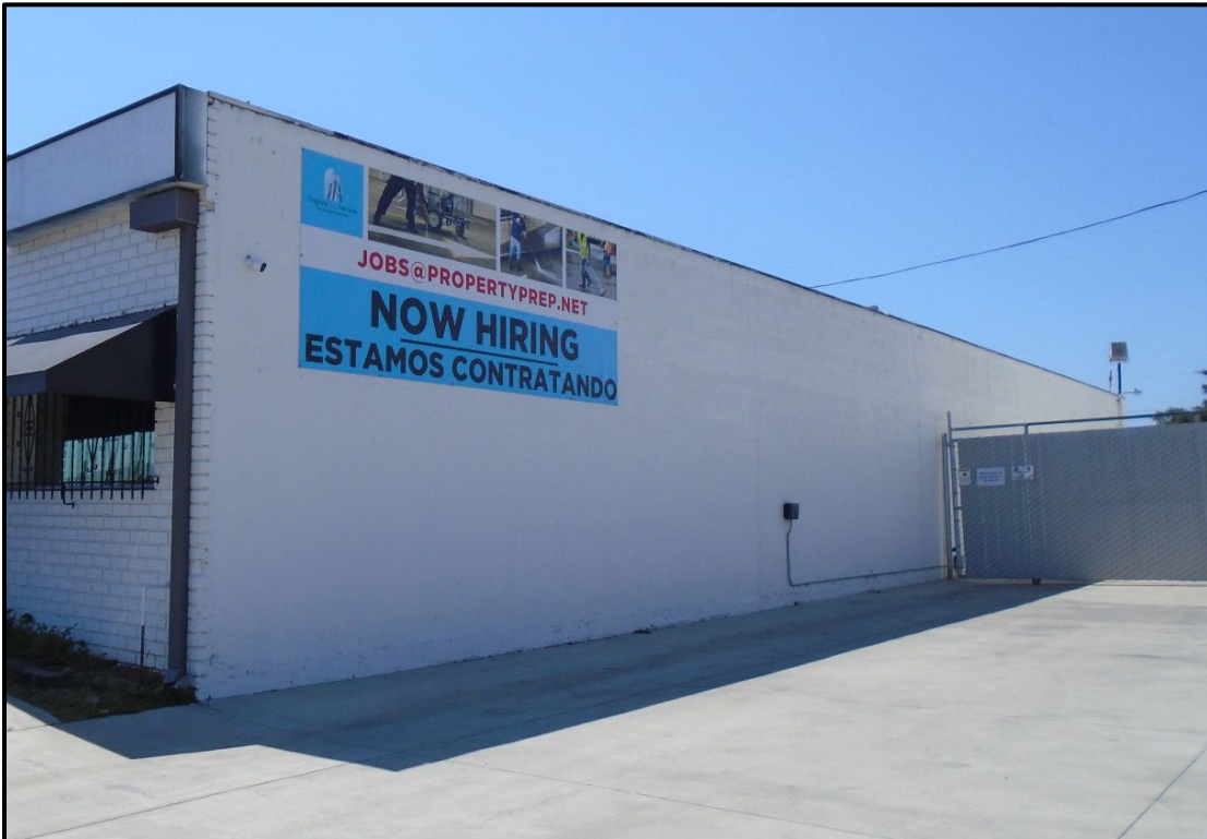
Figure 21. Building 3 (16835-16839 South Normandie Ave., APN 6106-030-015), north elevation, view southwest
