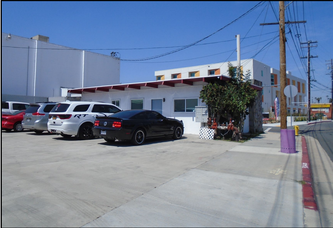
Figure 16. Building 2 (16829-16831 South Normandie Ave., APN 6106-030-011), south and east elevations, view northwest
