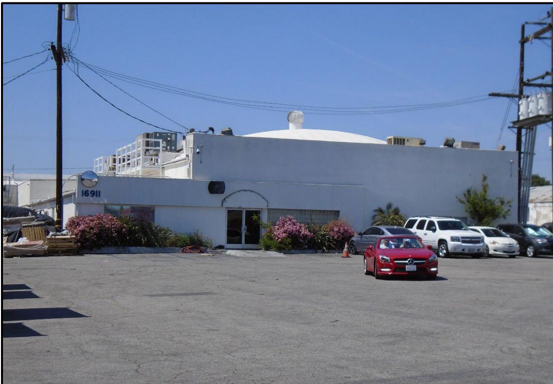
Figure 31. Building 5 (16911 South Normandie Ave., APN 6106-030-017), east elevation, view northwest
