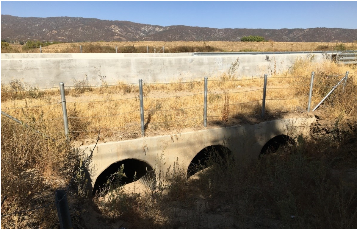
Photograph 6. Concrete drainage along SR 371 that connects to Cahuilla Creek, facing northeast.
