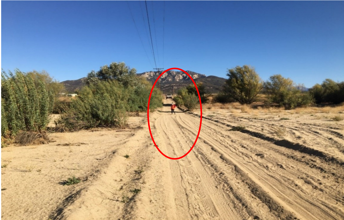
Photograph 7. Cahuilla Creek crossing. Note poles span the entire creek without contact.
