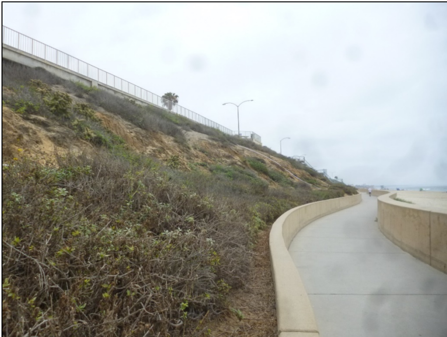
Photo 6. Typical view of footpath leading to beach, with retaining wall and sea wall to the left and right, respectively, of the path and native vegetation along the bluff. Date: July 10, 2018.
