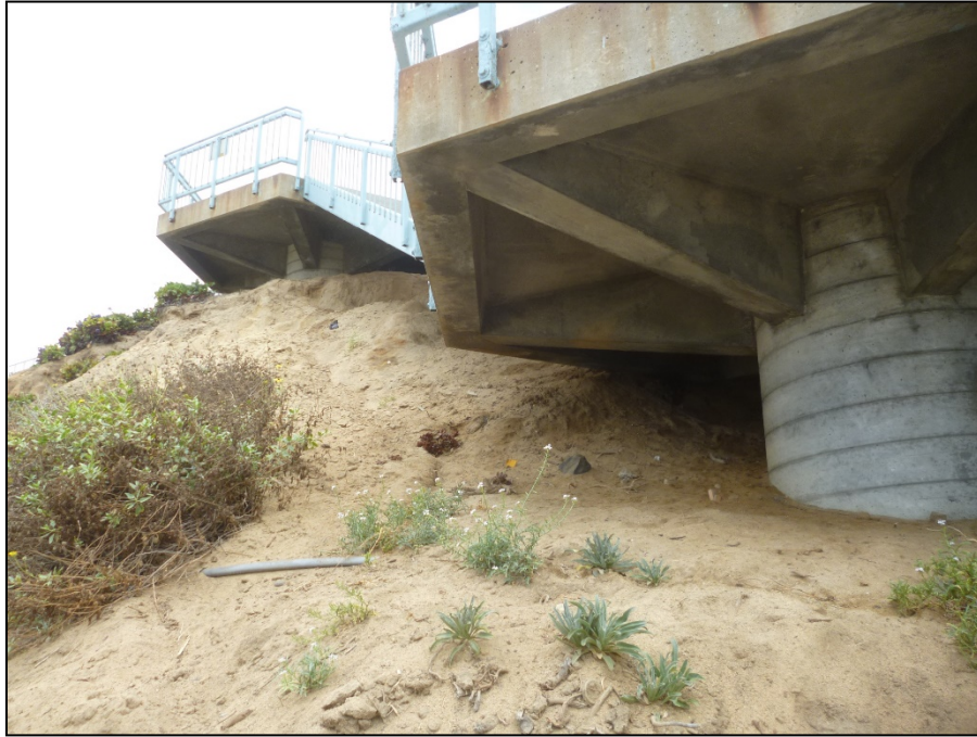
Photo 5. Underside of one of the stairways. Date: July 10, 2018.
