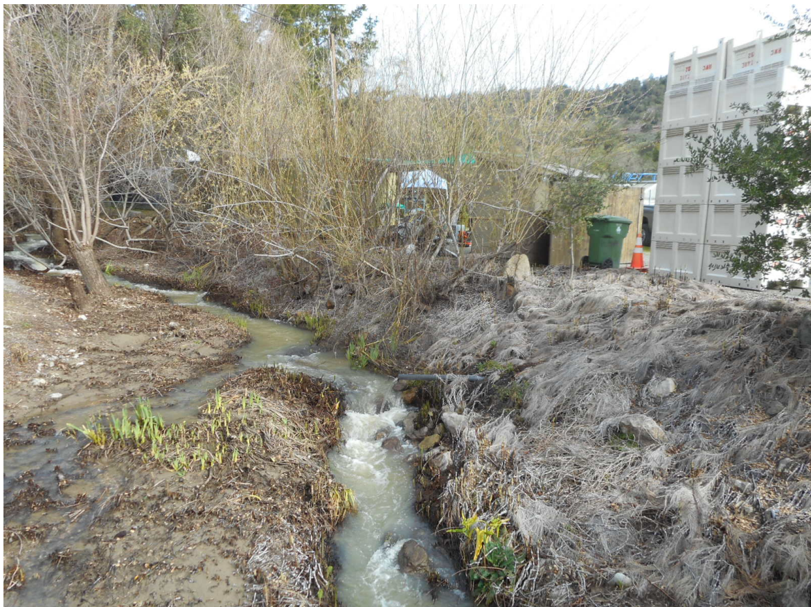
Photo 1. Revegetation site. Area of encroachment into 45-foot stream setback.
