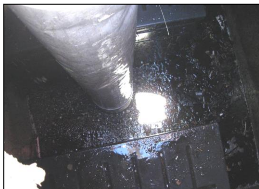
Removal of trash, sediment and debris.
