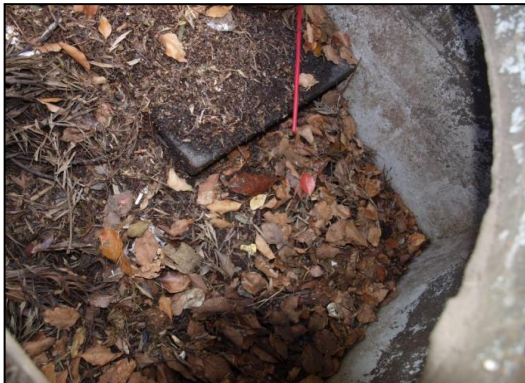
Removal of access hatch to gain access below.
