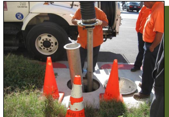
Insertion of vacuum hose into separation chamber.
