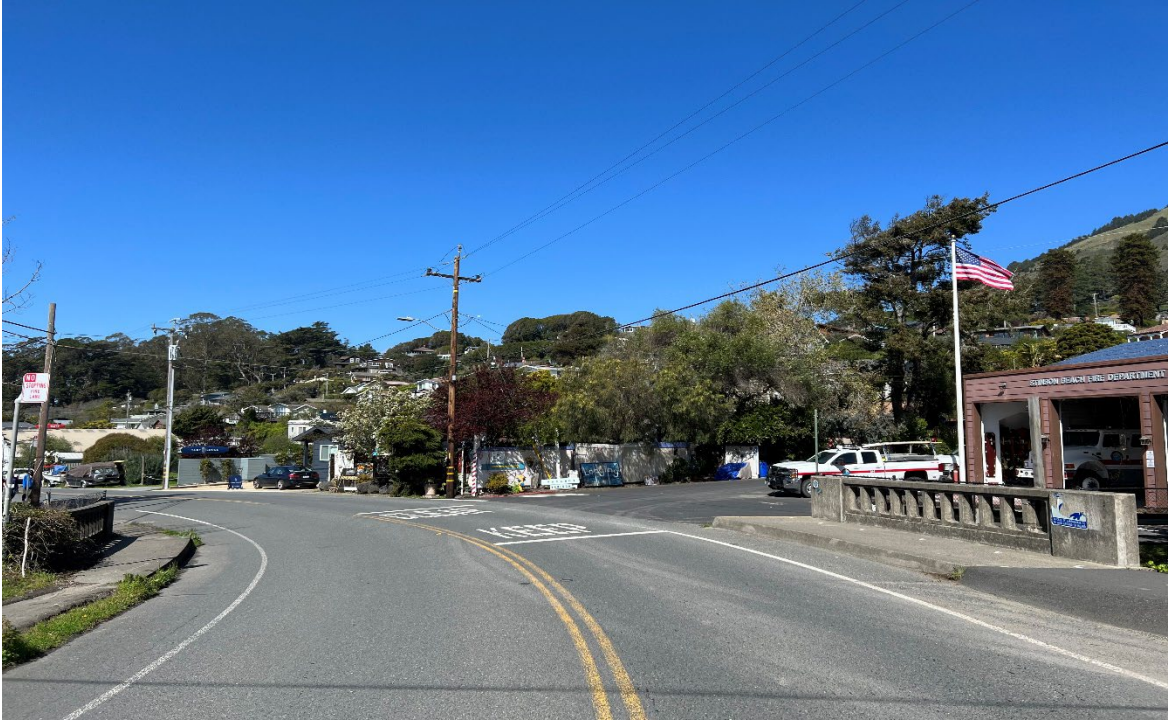
Figure 3.3.1-3. Eskoot Creek Bridge Existing Conditions Northbound View
