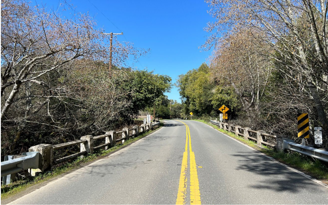
Figure 3.3.1-5. Olema Creek Bridges Existing Conditions Northbound View
