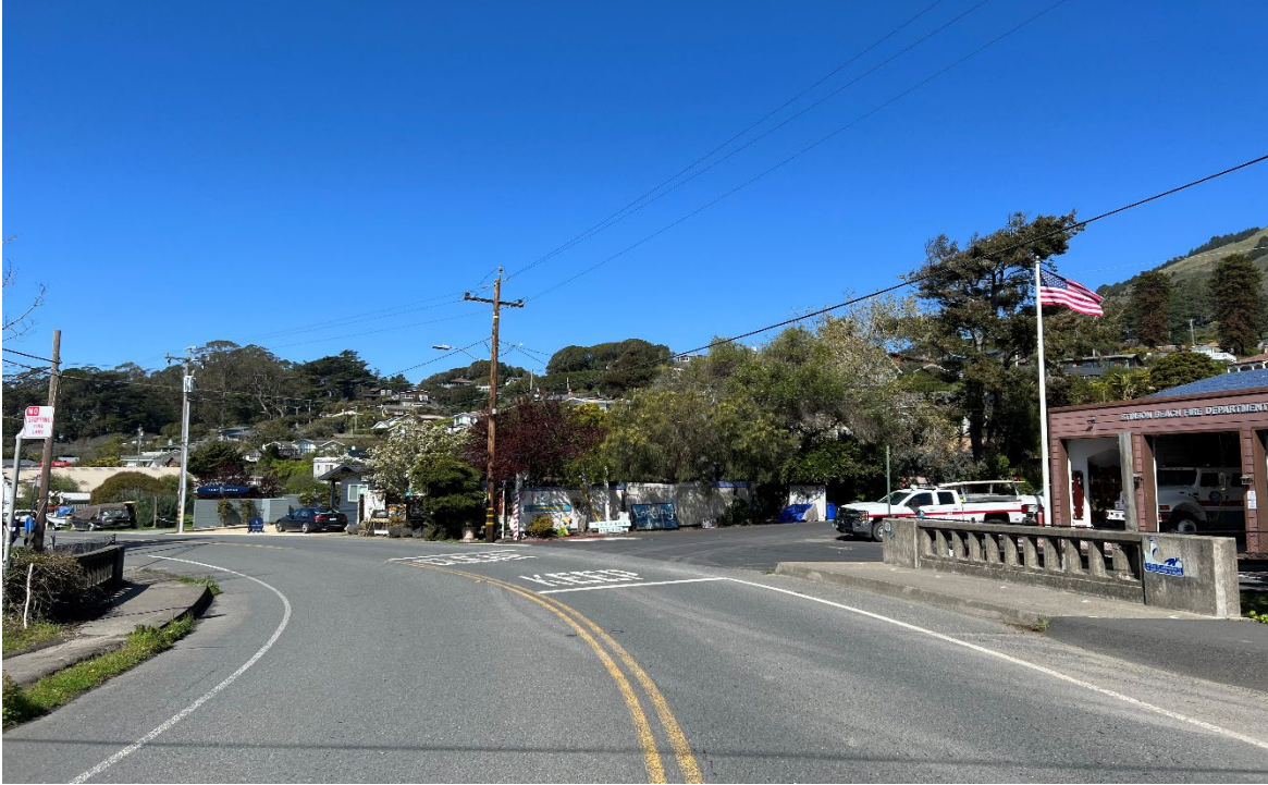
Figure 3.3.1-3. Eskoot Creek Bridge Existing Conditions Northbound View
