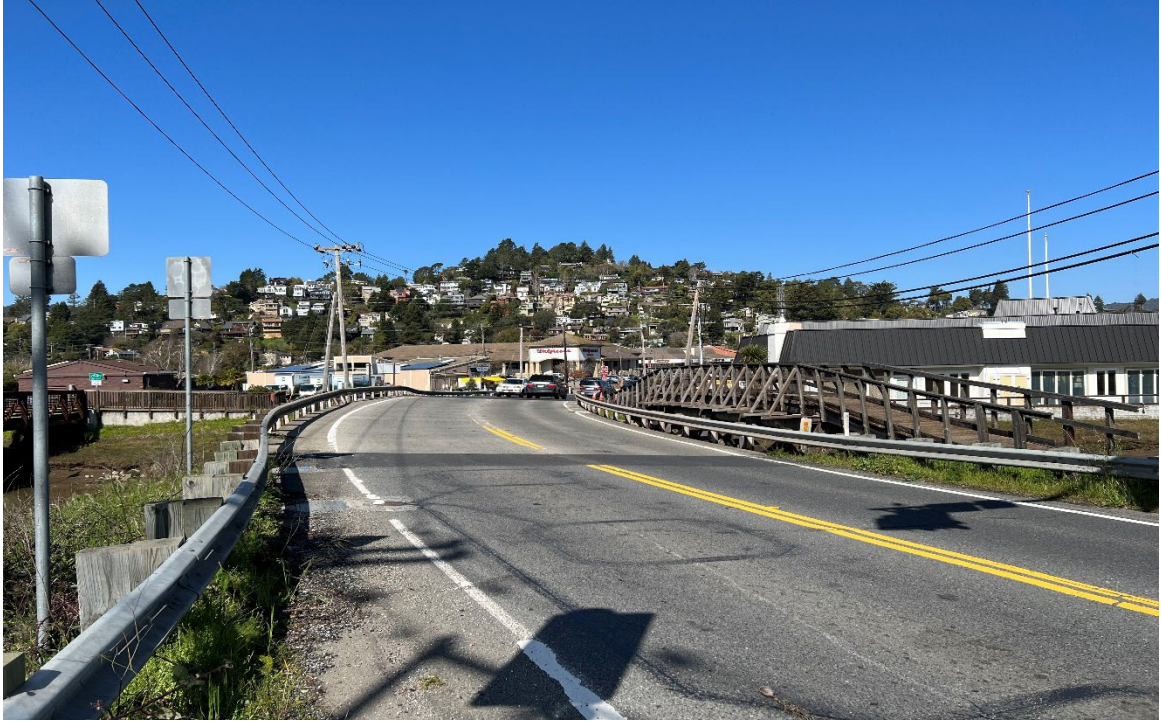
Figure 3.3.1-1. Coyote Creek Bridge Existing Conditions Northbound View
