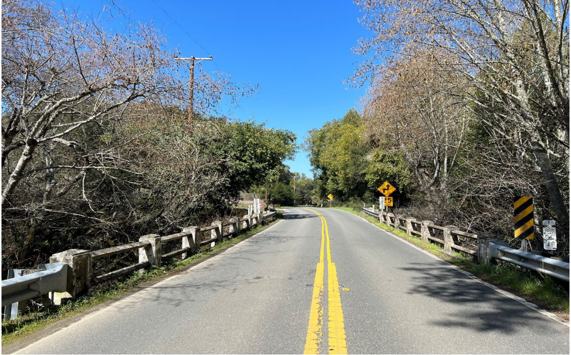
Figure 3.3.1-5. Olema Creek Bridges Existing Conditions Northbound View
