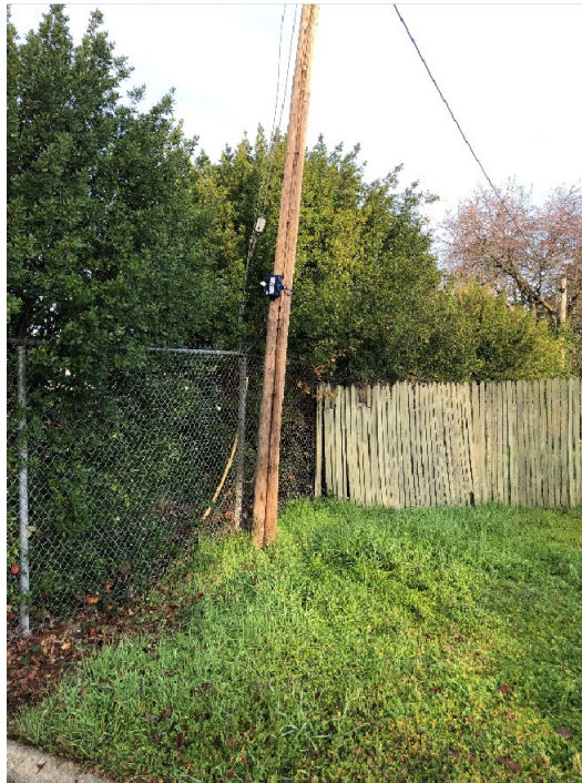
SLM attached to a telephone pole at the dead end of Y Street.
