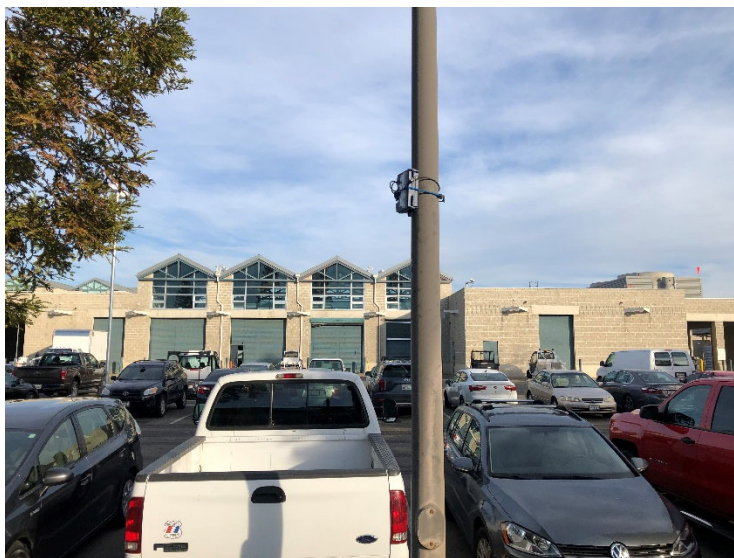
Looking North at motor pool facility.
