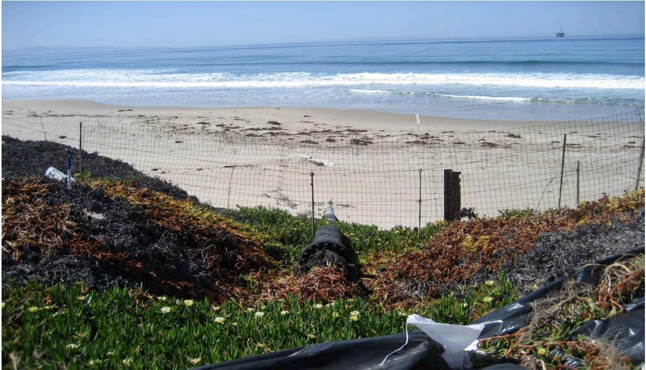
**Photo 2.** View of the Loading Line at the bluff face, looking southwest. The fence in the foreground and white sign at the high tide line marks the Sensitive Species Exclusion Zone boundaries. Note concrete pipeline support exposed on beach inside the exclusion zone.
