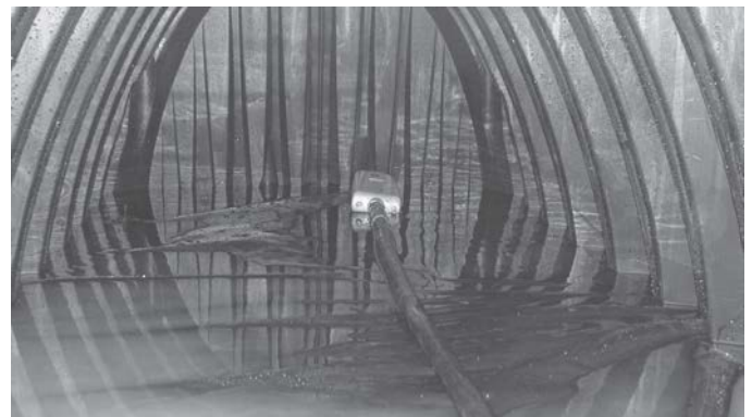
Figure 1. Containment Row shown with high pressure cleaning nozzle.
