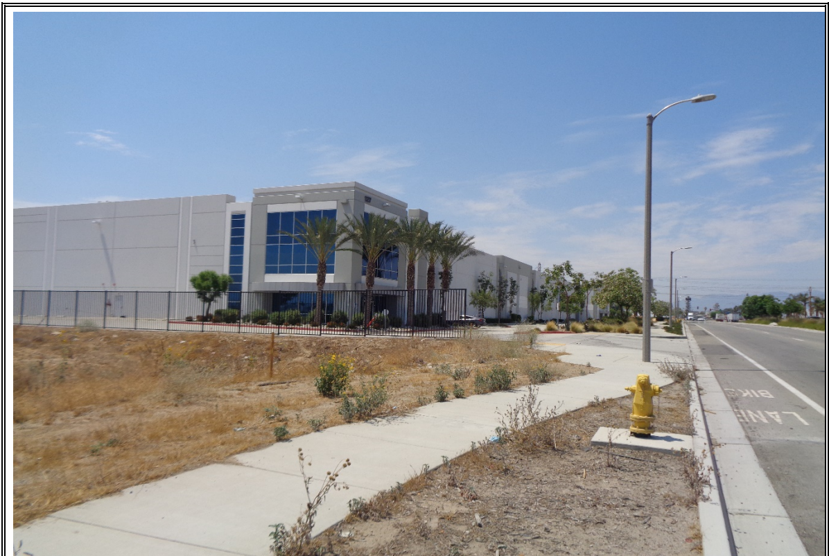
Photograph Number 15: Commercial/industrial to the further north.
