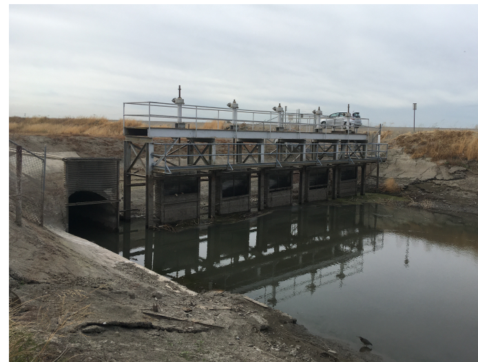
Photo 6: Looking at Dam from Staging Area
