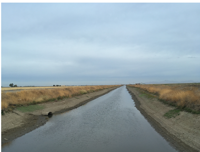
Photo 7: Top of Dam Looking NE at Irrigation Canal
