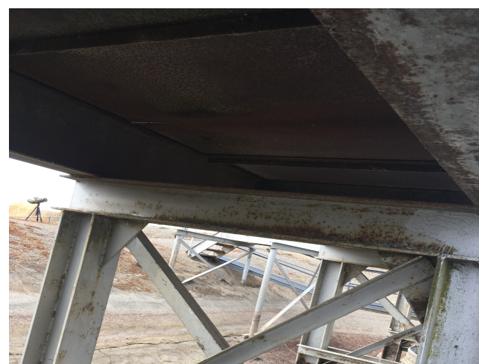
Photo 8: Underside of Metal Dam Structure No Swallow or Bat Nests
