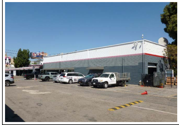
Building A, south façade, view northwest (ARG, 2022)
