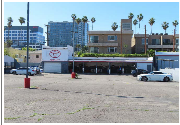
Car Wash Canopy, view south (ARG, 2022)
