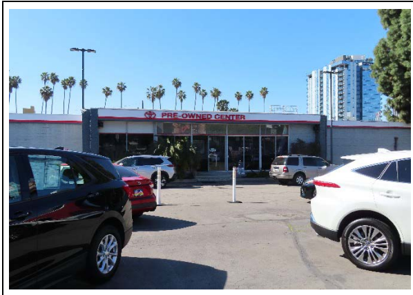
Service Bay A, detail of entrance on north façade, view southwest (ARG, 2022)
