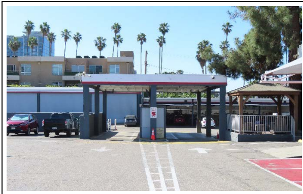
Entrance Canopy, view south (ARG, 2022)
