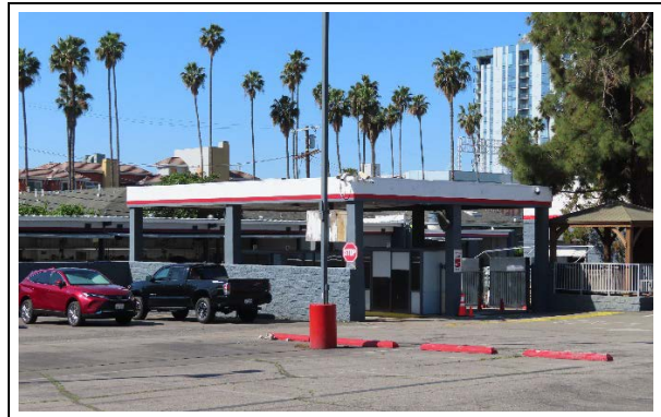
Entrance canopy, view southwest (ARG, 2022)
