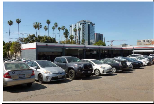
Service Bay C, view southwest (ARG, 2022)
