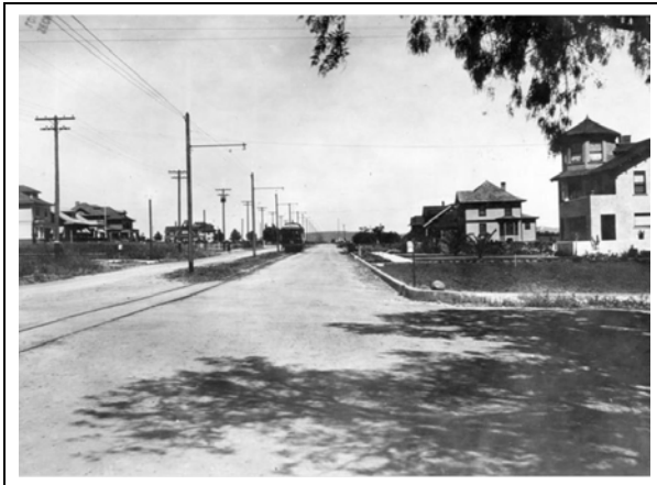
Hollywood Blvd, looking east from Gower St, ca. early 1900s. The subject site, then-developed with houses, is pictured at right (Los Angeles Public Library)
