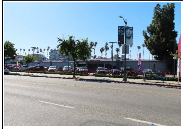
Service Bay A, primary/north façade, view southeast (ARG, 2022)
