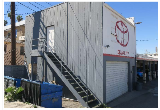
Car wash canopy, view southwest. Note exterior stair and upper-story entrance (ARG, 2022)
