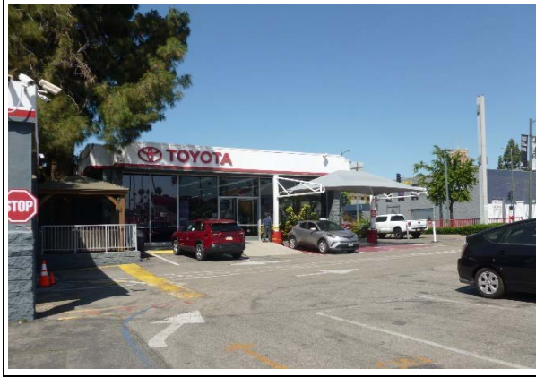
Building A, east façade, view northwest (ARG, 2022)
