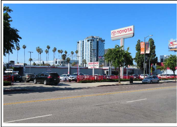
Service Bay A, primary/north façade, view southwest (ARG, 2022)
