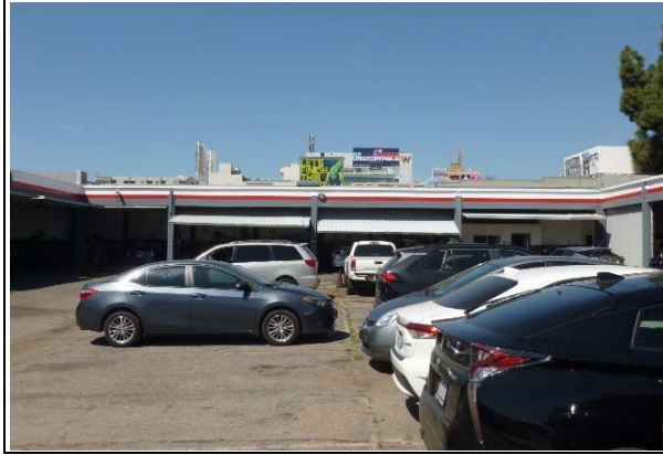
Service Bay B (at center rear), view west (ARG, 2022)
