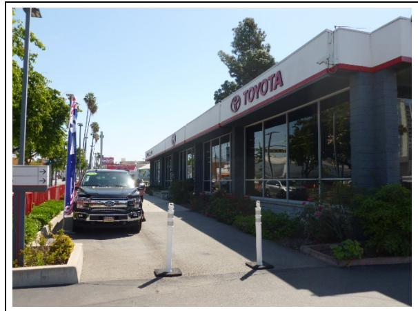
Building A, primary/north façade, view southeast (ARG, 2022)
