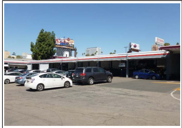
Service Bay A, south façade, view northwest (ARG, 2022)
