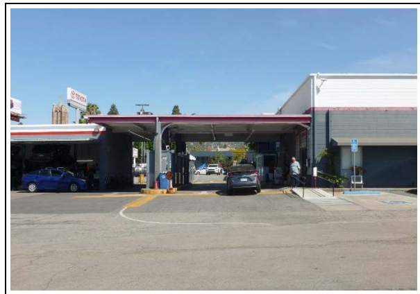
Canopy structure appended to the west façade of Building A (right), view north (ARG, 2022)
