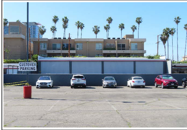
Service Bay E, view south (ARG, 2022)
