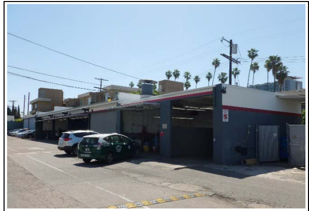
Service Bay D, view southeast (ARG, 2022)
