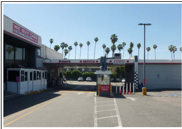
Canopy structure appended to the west façade of Building A (left), view south (ARG, 2022)
