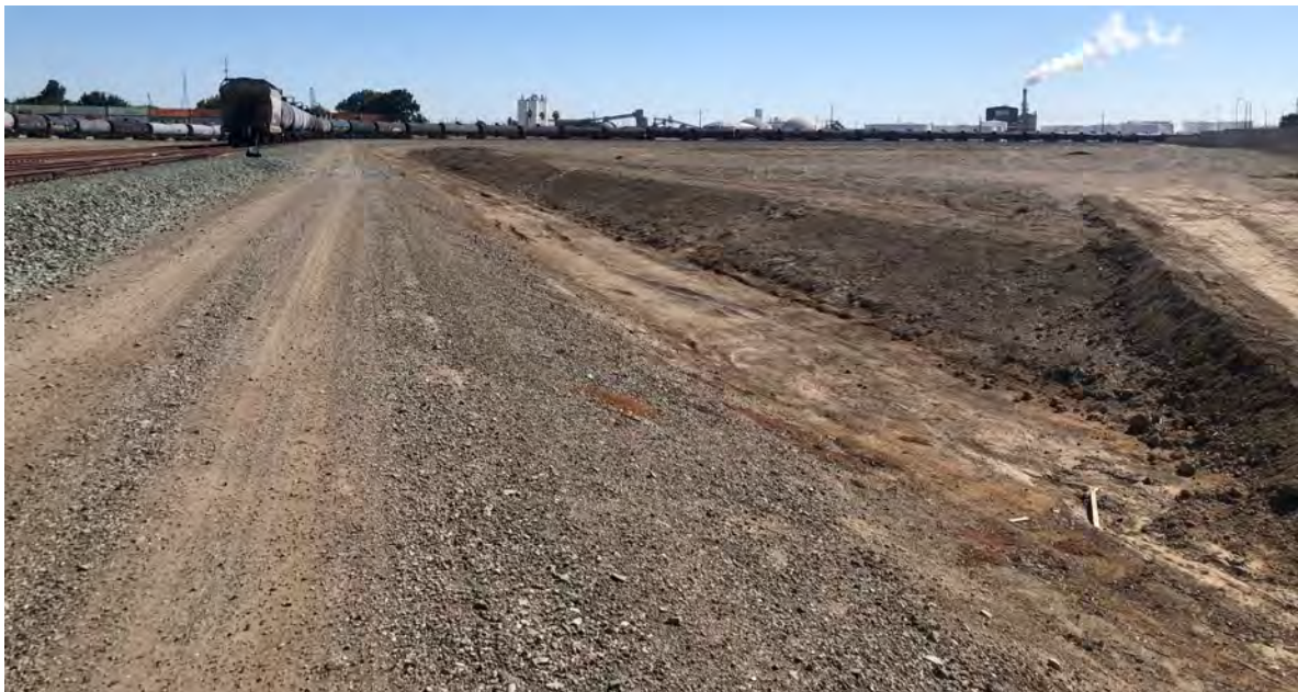
Photograph 7 Drainage Ditch on Project Site, August 2022
