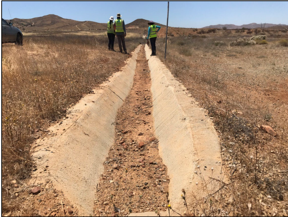
Photo 3: Concrete drainage culvert along North Project boundary, facing West
