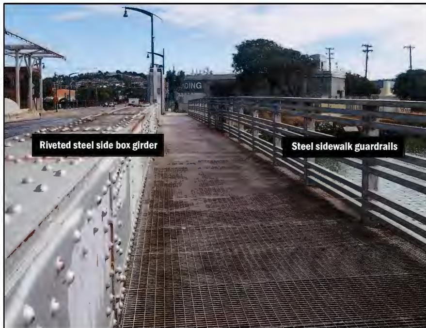
Figure 4.B-2 Above-Deck Character-Defining Features, Facing South
