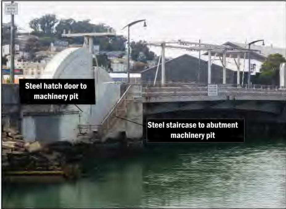
Figure 4.B-3 Character-Defining Steel Staircase Leading to Abutment Machinery Pit and Sidewalls of Concrete Abutments, at Southeastern Corner Leading to Steel Hatch Door, Facing Northwest
