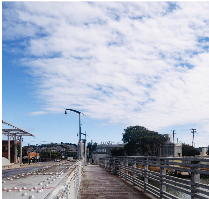
Figure 4 Existing View from Islais Creek Bridge Facing South
