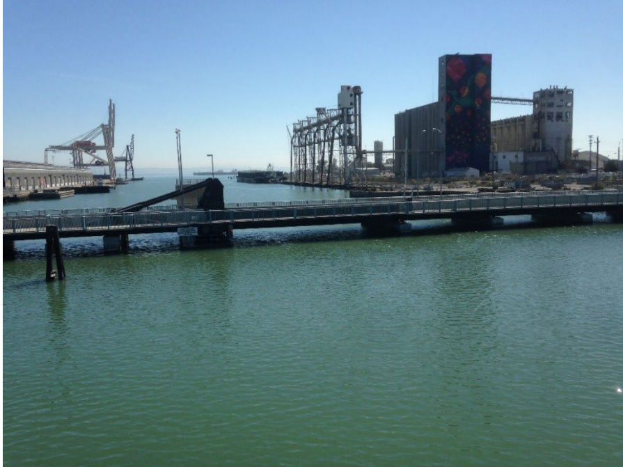
Figure 1 Existing View from Islais Creek Bridge Facing East
