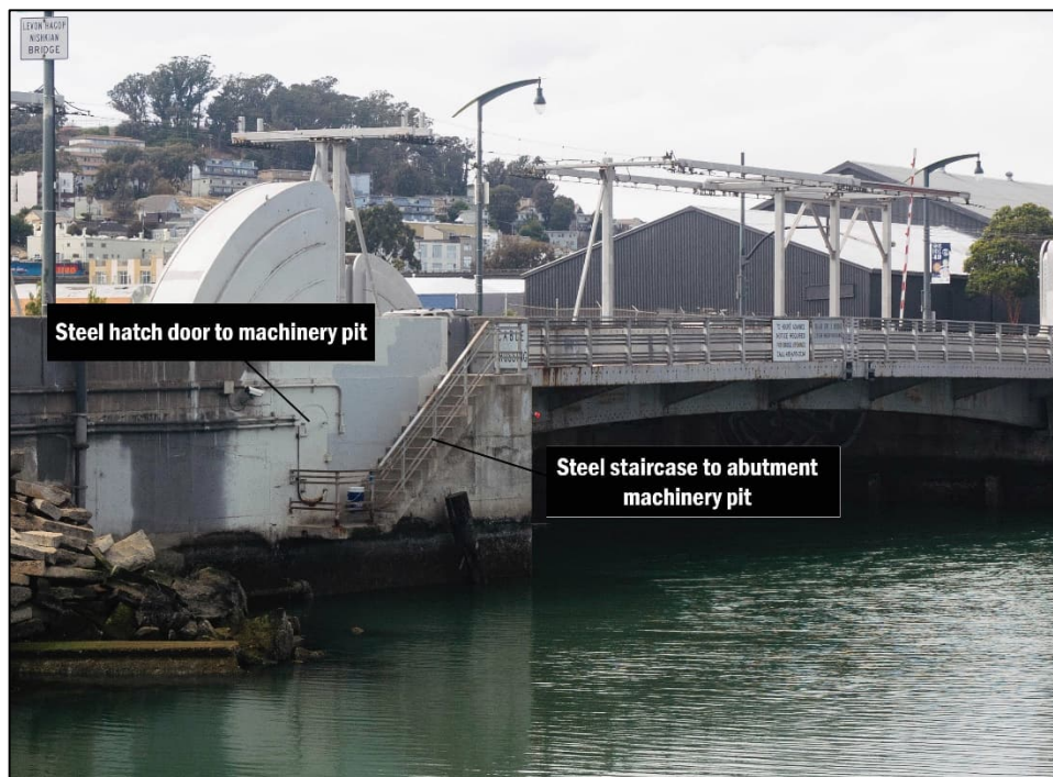
Photograph 3. Character-defining steel staircase leading to abutment machinery pit and sidewalls of concrete abutments at southeast corner leading to steel hatch door, facing northwest
