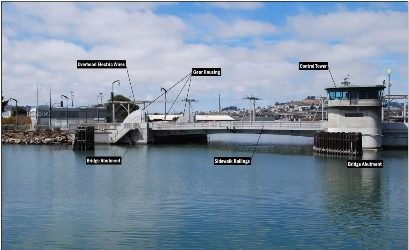
Figure 2. Islais Creek Bridge East Elevation
