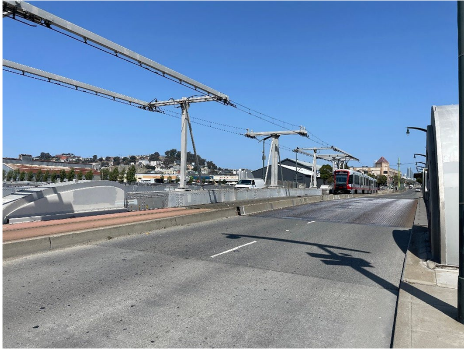
Figure 3 Existing View from Islais Creek Bridge Facing North
