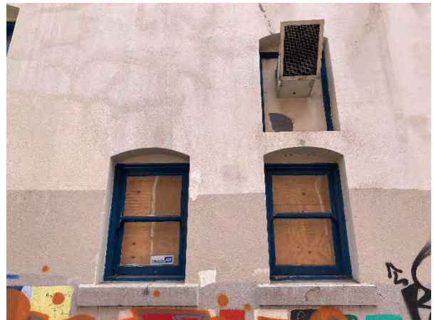
Figure 52: Smaller segmental arched windows along the west façade, looking east.
