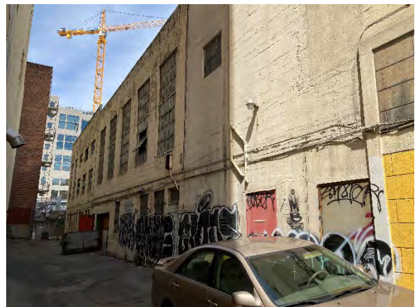
Figure 24: Oblique view of the alley behind the subject buildings, facing west.
