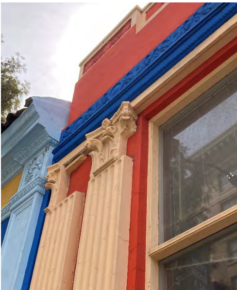
Figure 45: Detail of partially intact capitals above the east pair of pilasters.
