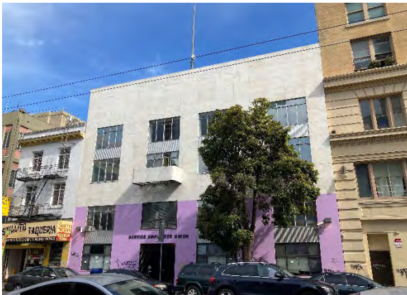
Figure 17: Moderne style building at 240 Golden Gate Avenue.
