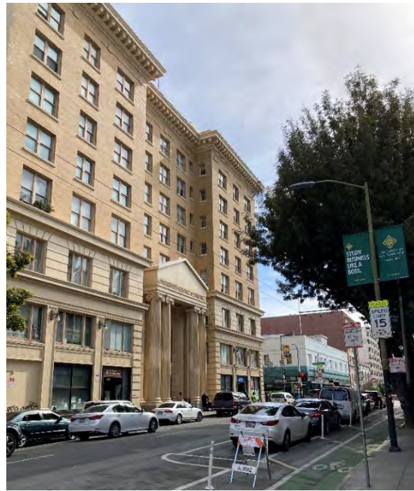
Figure 16: Y.M.C.A Building at 210-220 Golden Gate Avenue, opposite the subject buildings.
