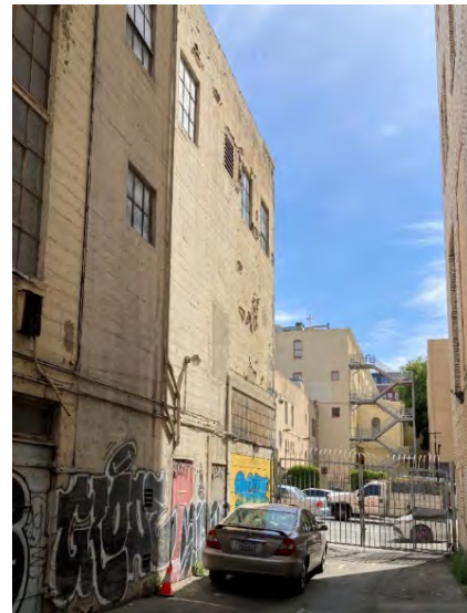
Figure 29: Rear, alley-facing façade, looking northwest.
