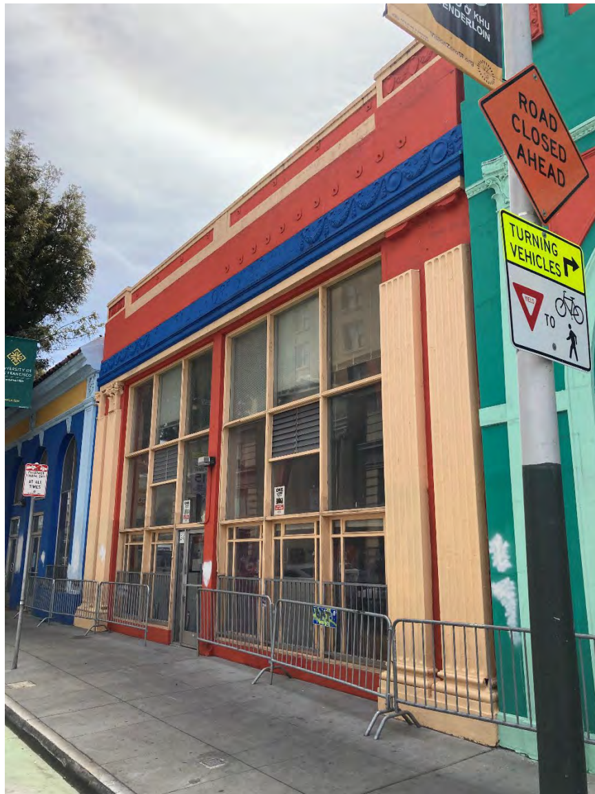
Figure 44: Primary (north) façade of 241-243 Golden Gate Avenue, looking southeast.
