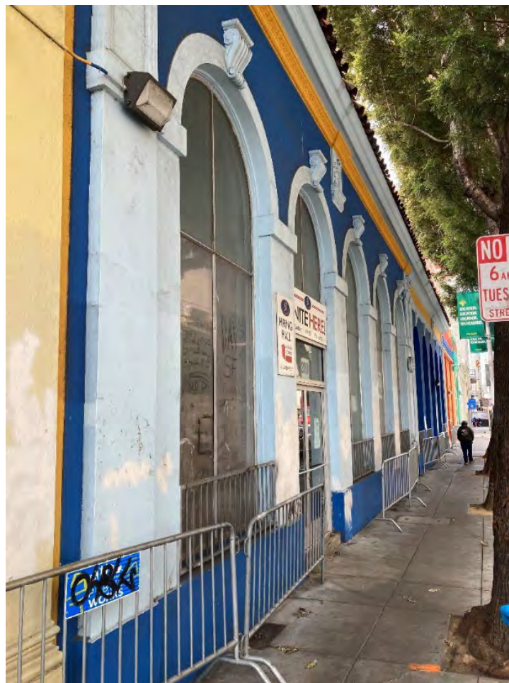
Figure 36: Primary (north) façade of 209 Golden Gate Avenue, looking west.
