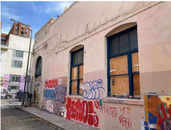
Figure 51: Segmental arched double windows at the west façade, looking north.
