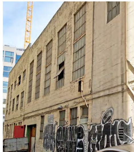
Figure 38: Rear façade of 209 Golden Gate Avenue, looking northwest.
