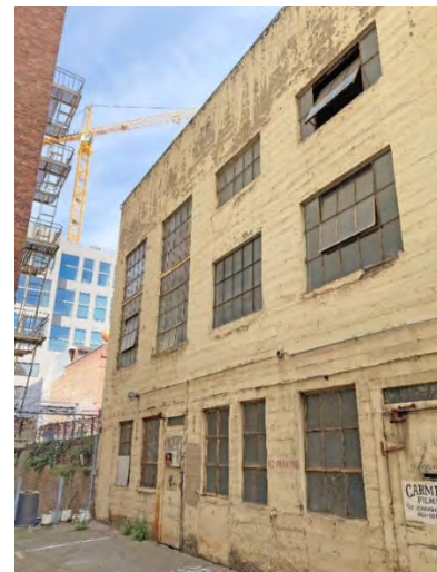
Figure 42: Rear façade of 215-229 Golden Gate Avenue, looking northwest.
