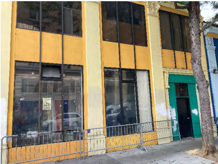
Figure 28: Primary façade, looking southwest.
