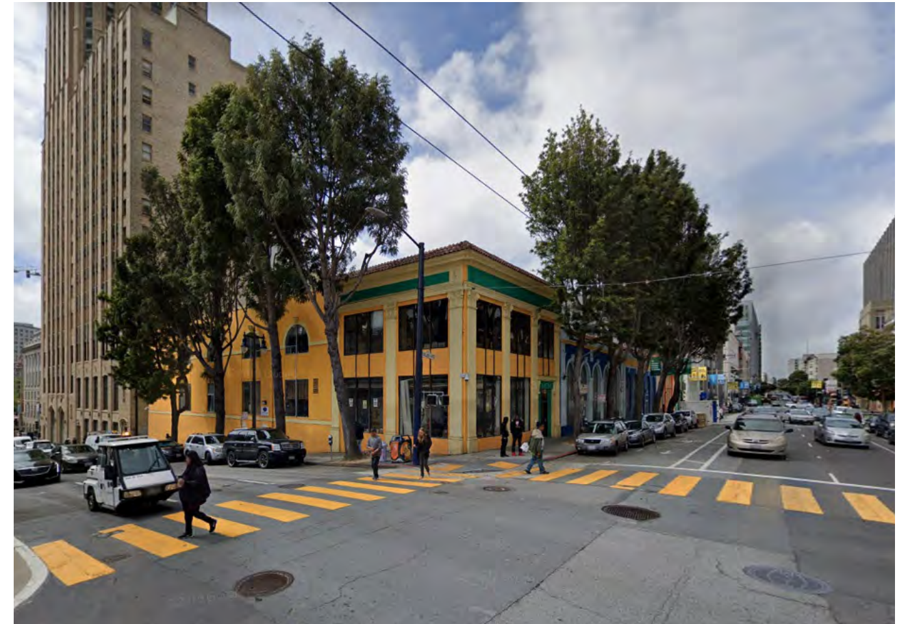
Existing Local 2 buildings (credit Google Street View) - Proposed Project Site
