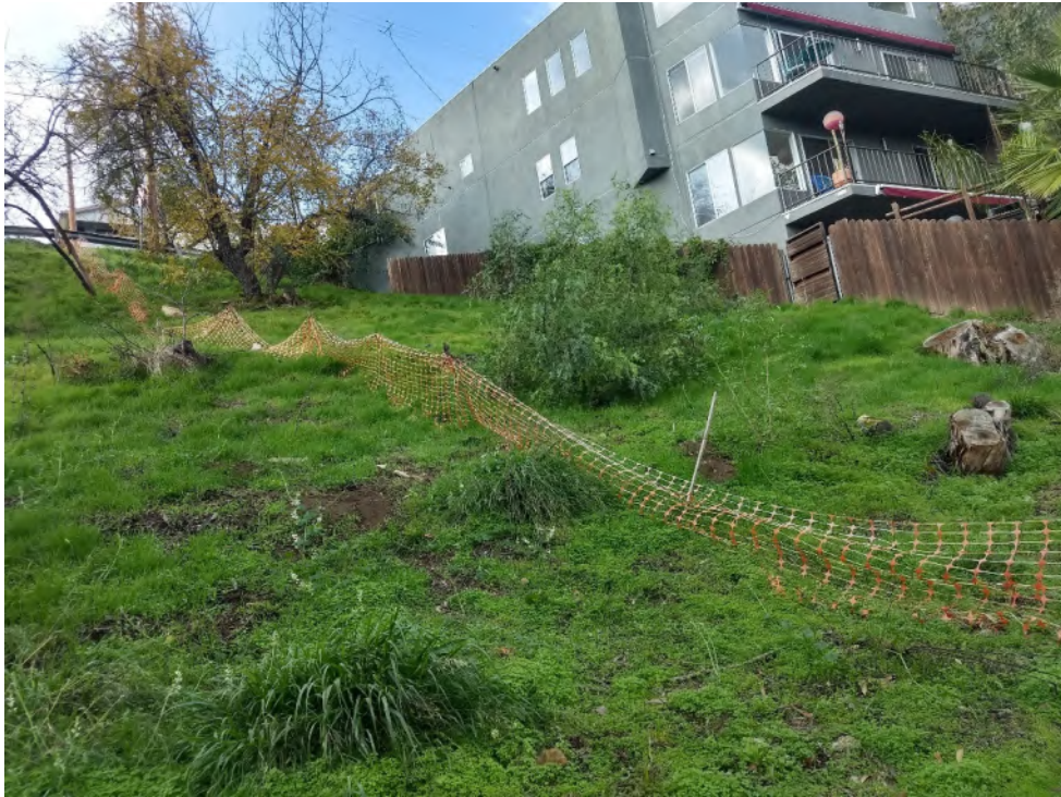
Image 3: Depicts the trees on 469 Del Norte and the northern adjacent residence. Photo taken from north-central portion of the survey area facing west.
