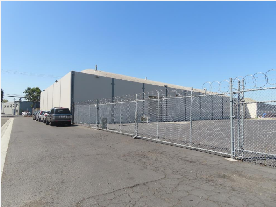
Photograph 2. Rear (north) an east elevations 985 O'Brien Drive. View looking southwest (IMG_0857).
