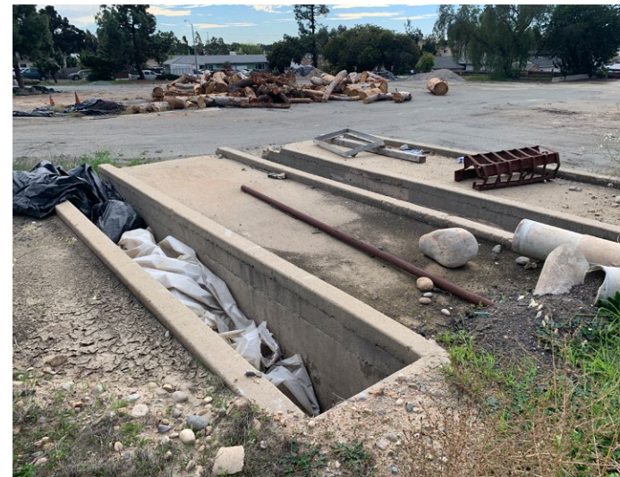
Remaining foundations from County Road Station
