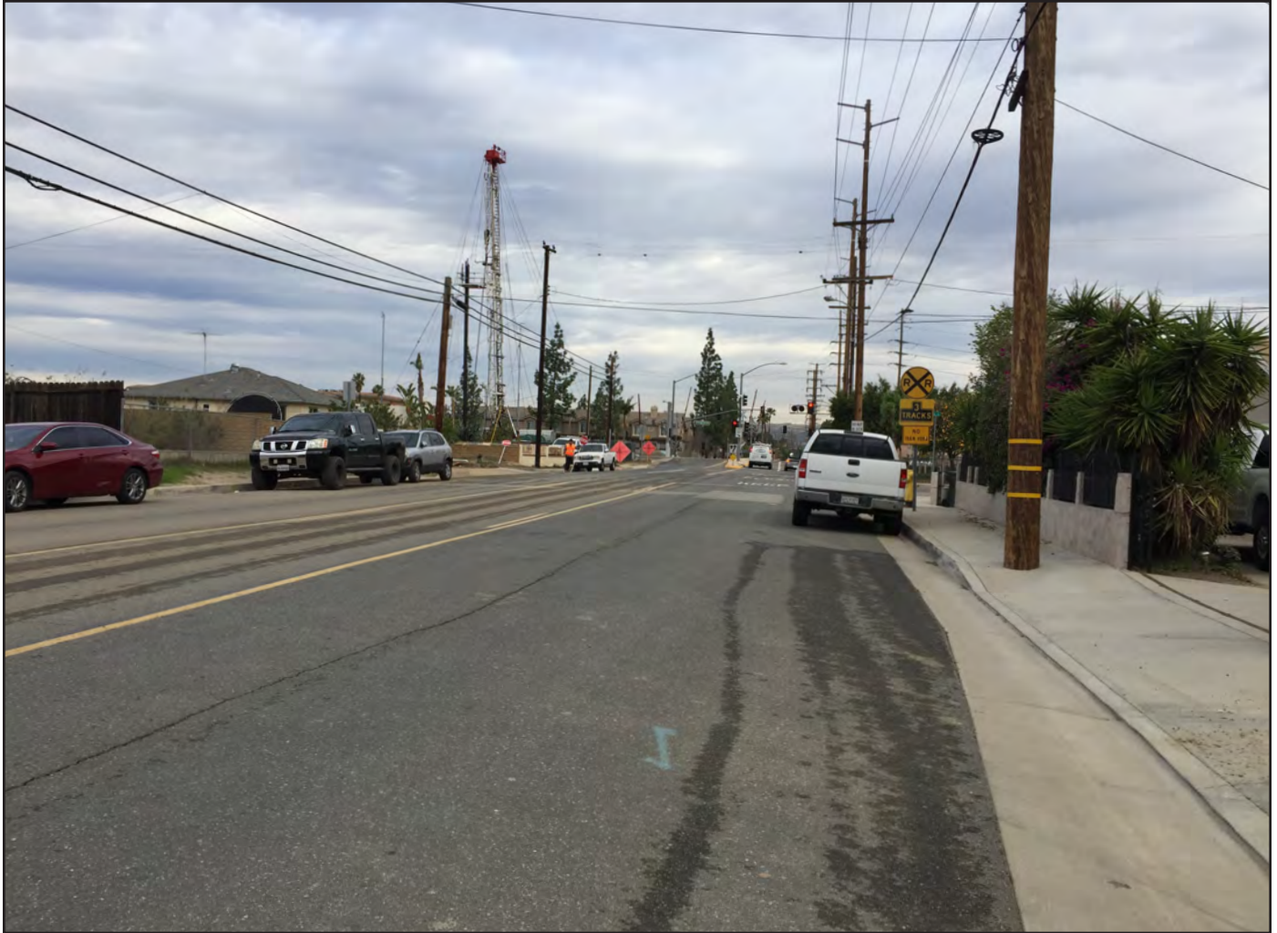
PHOTO 10 At Van Buren - North View
