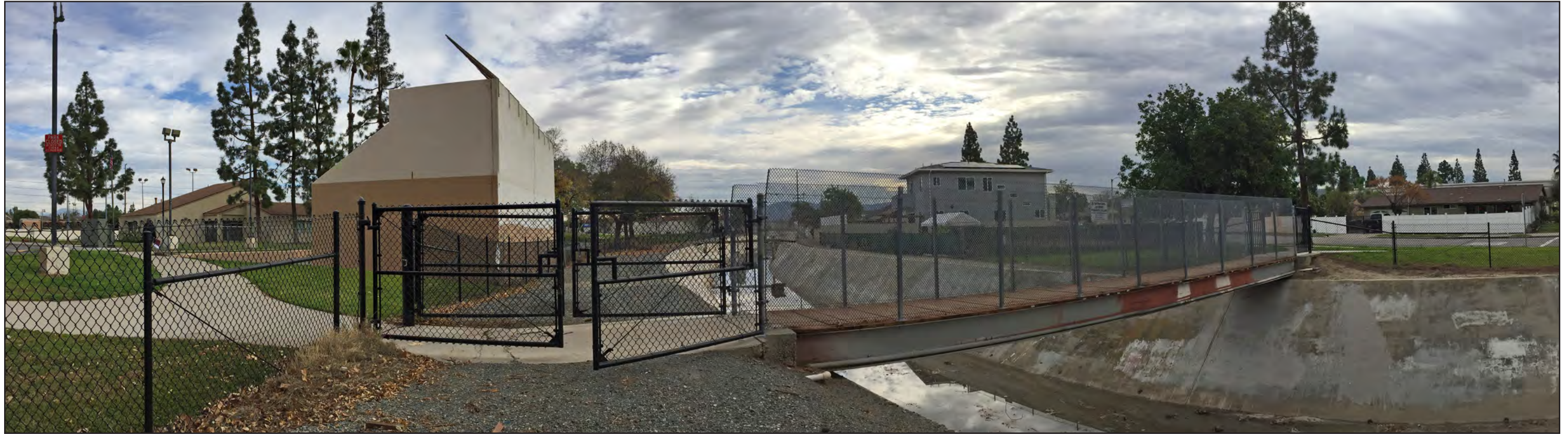
PHOTO 17 At Maria Ave Crossing - West View
