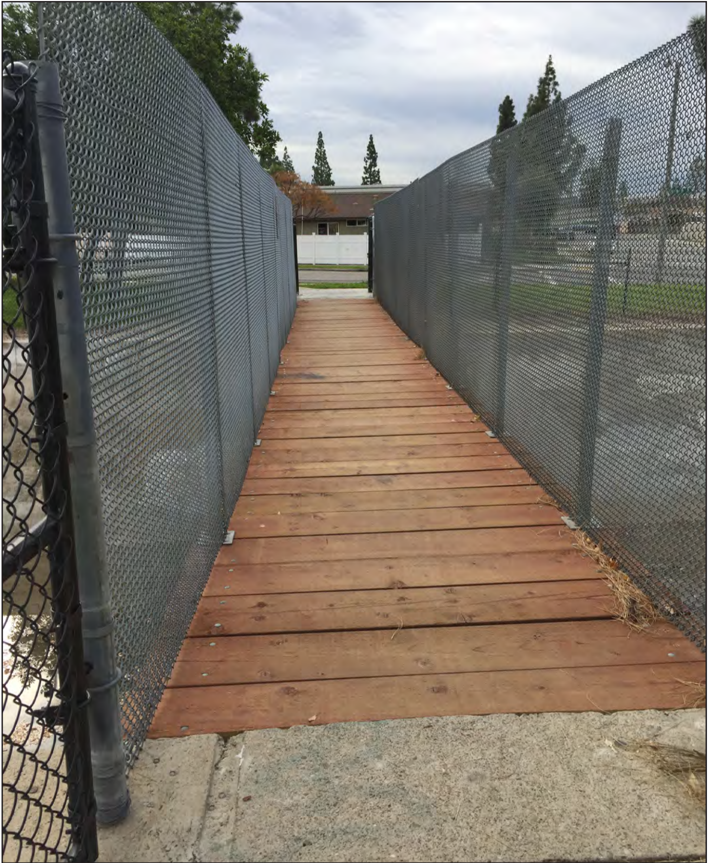
PHOTO 18 At Maria Ave Bridge Crossing - South View
