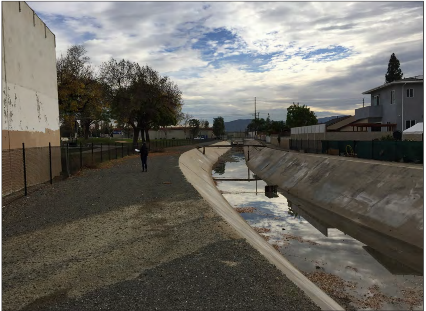
PHOTO 20 Maria Bridge Crossing-ParqueNiños - East View
