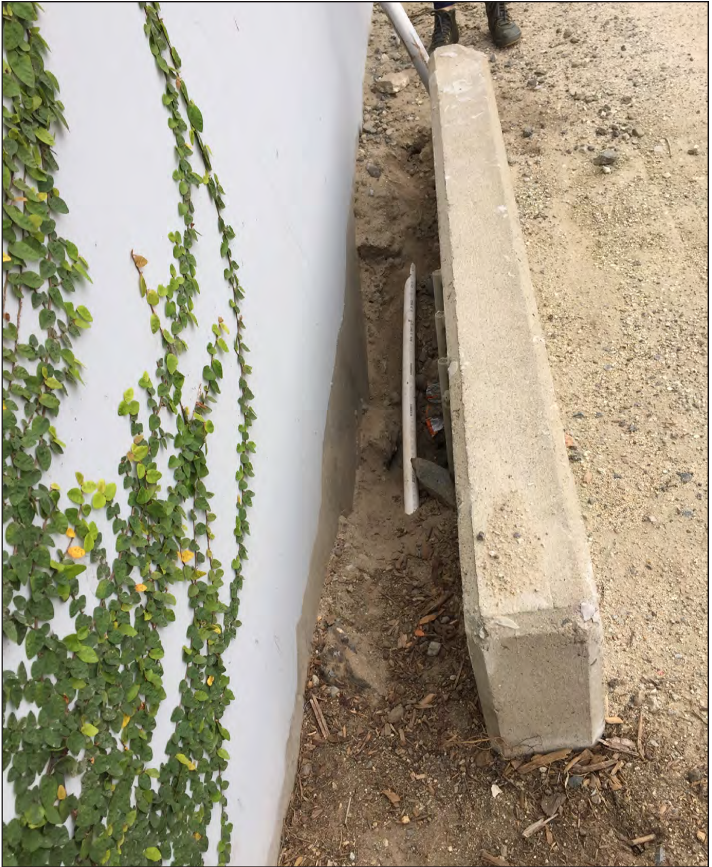
PHOTO 40 At Veterans Village - View of Infrast-drainage
