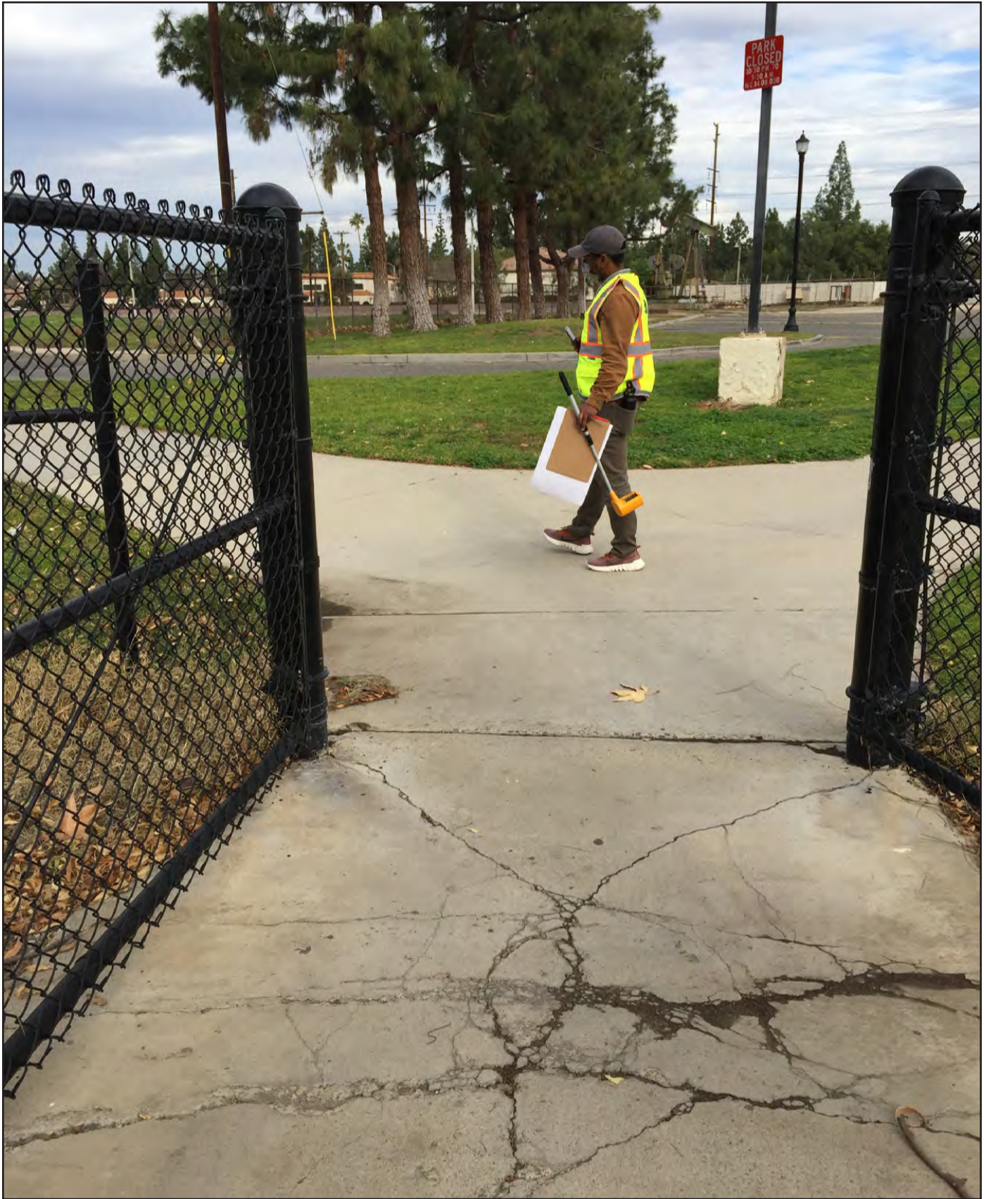
PHOTO 19 At Maria Ave Bridge Crossing - North View
