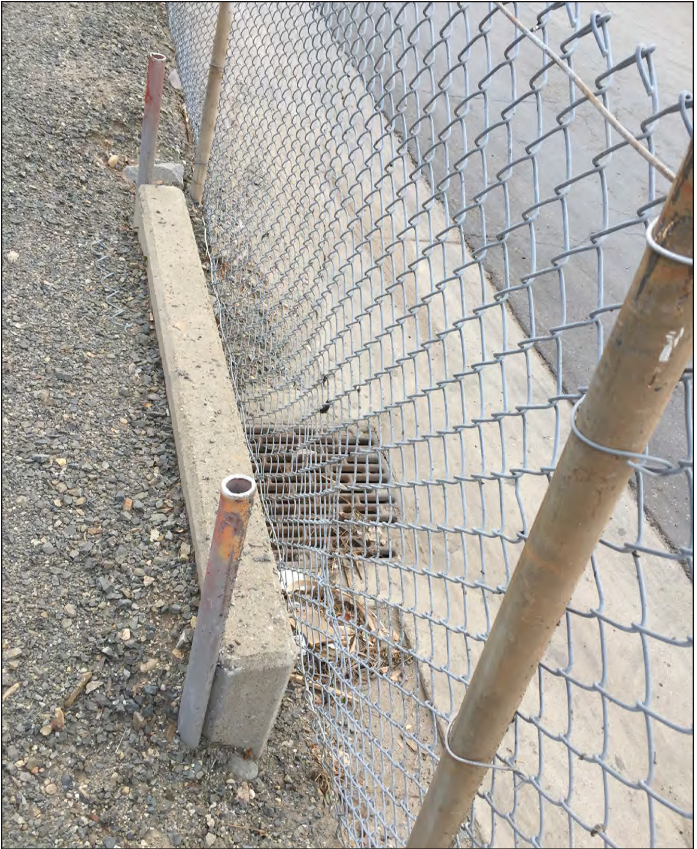
PHOTO 6 BNSF-Van Buren View - Ex Infrac Drainage
