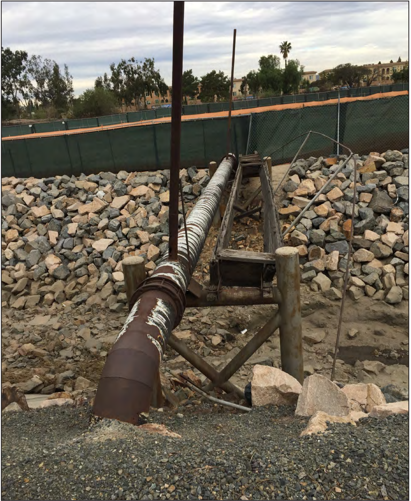
PHOTO 5 BNSF-Van Buren View - Ex Infrastructure
