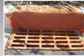
Combination inlet with magnetic rear guard attachment
