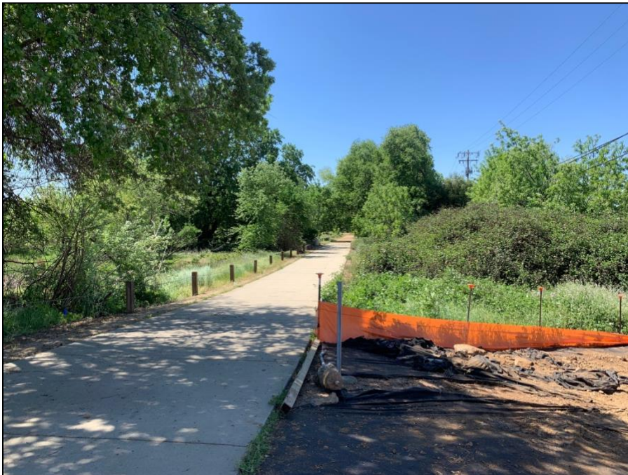
Figure 10. Pedestrian walkway parallel to Auburn Ravine, view southwest
