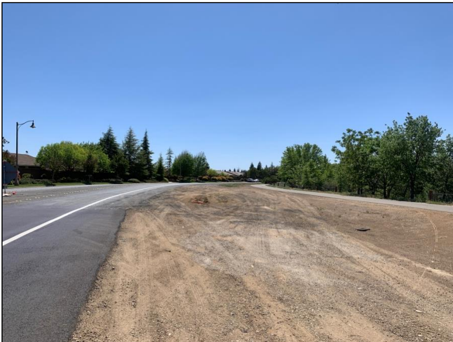
Figure 8. McBean Park Drive at Ferrari Ranch Road, view southwest
