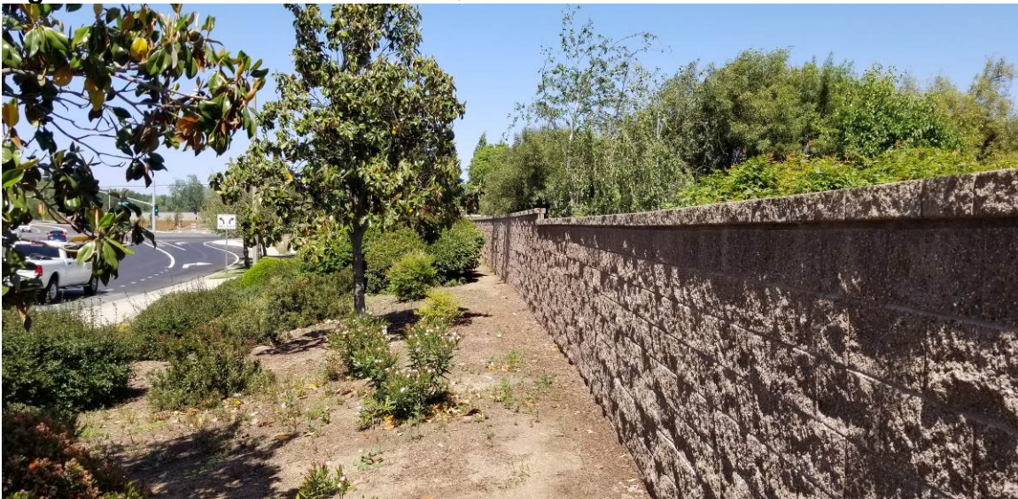
Figure 5-1. Barrier in Southeast Quadrant of Intersection
