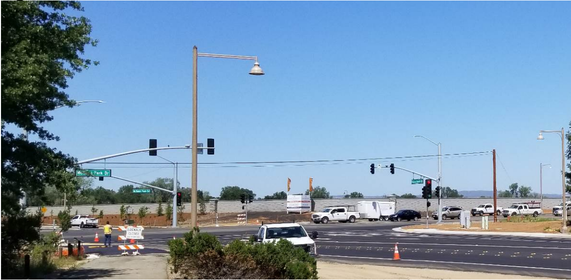
Figure 5-2. Barrier in Northeast Quadrant of Intersection
