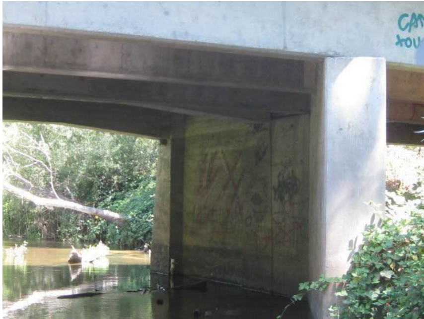
Photograph 11: Under McBean Park Drive Bridge. Photograph taken August 15, 2014 by A. Rich.
