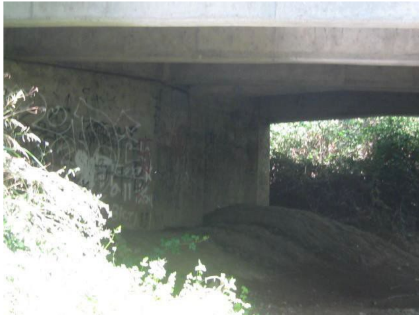
Photograph 12: Under McBean Park Drive Bridge. Photograph taken August 15, 2014 by A. Rich.
