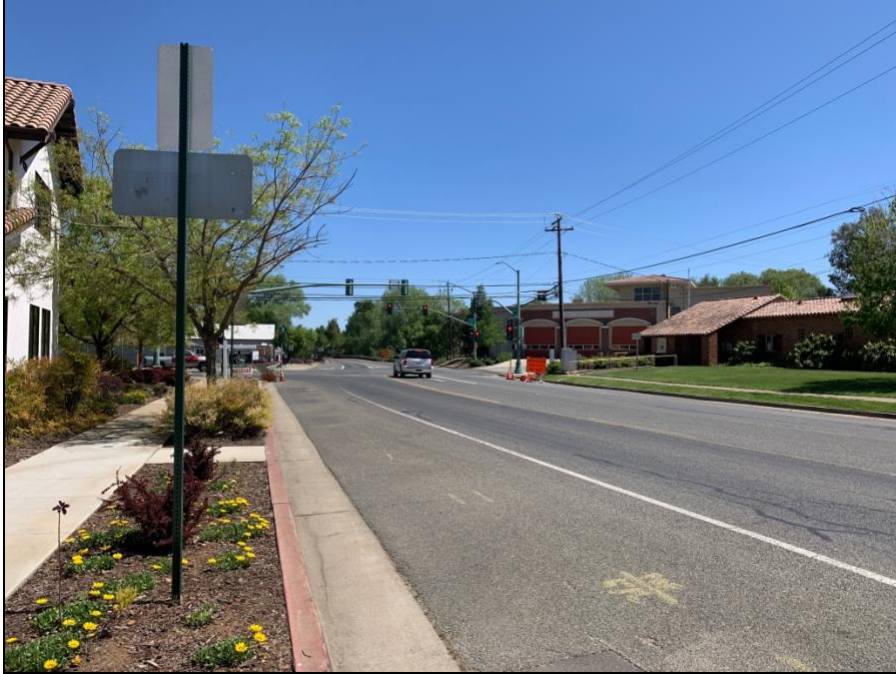
Figure 7. Overview of McBean Park Drive from the corner of 'A' Street, view southeast
