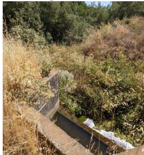
P04 – Culvert (C01) and diversion channel (OW03) looking northeast
