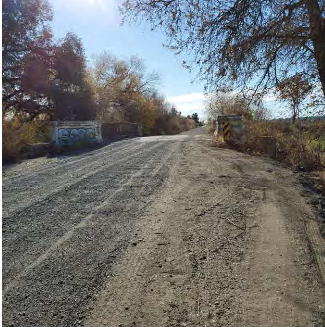
Figure 5. Overview of the bridge approach, viewing south
