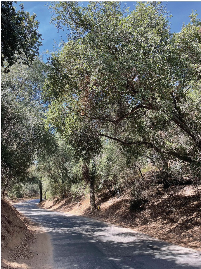
Southwest View - South End of Pipeline 6
