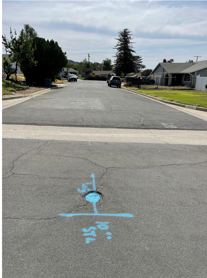
East View of Bing Place
