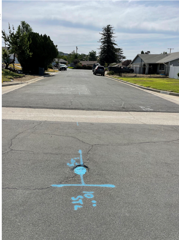
East View of Bing Place
