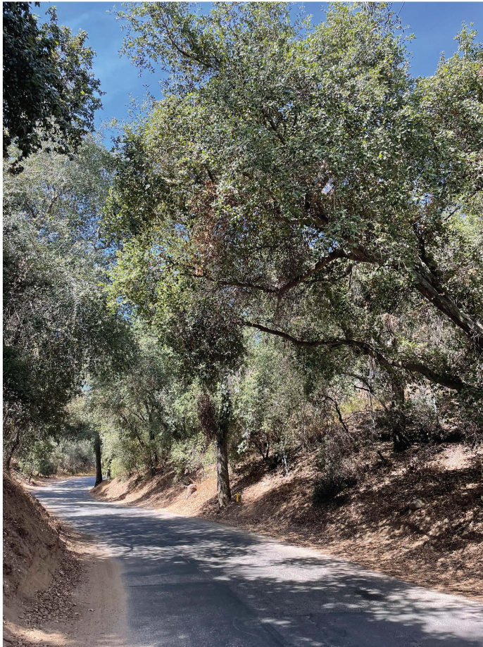
Southwest View - South End of Pipeline 6
