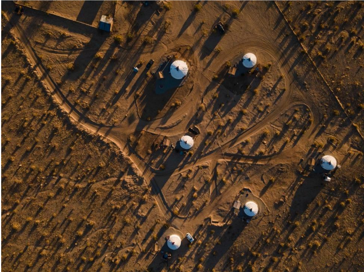
Photo 1: Aerial view of easterly parcel showing the existing Yurt configuration
