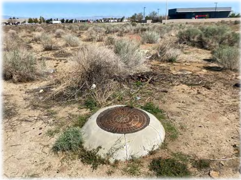
23. View of sewer manhole lid south of the Forbes Street cul-de-sac.
