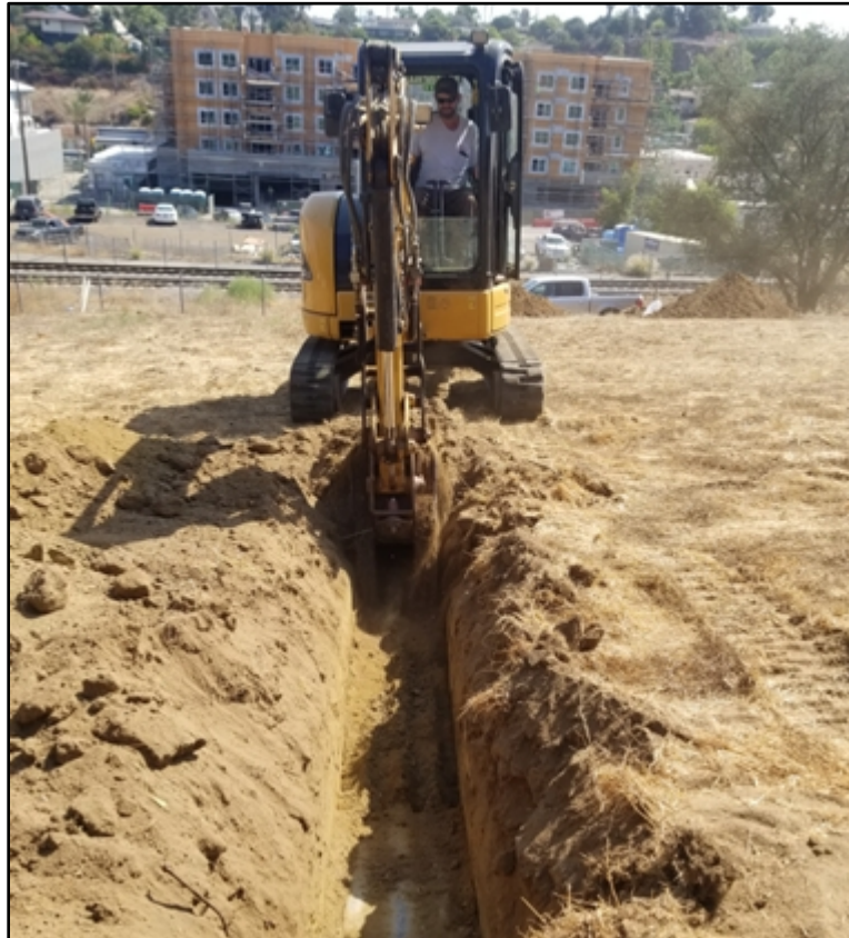
Figure 3-2. Test Pit Excavation (TP-5, August 2021)
